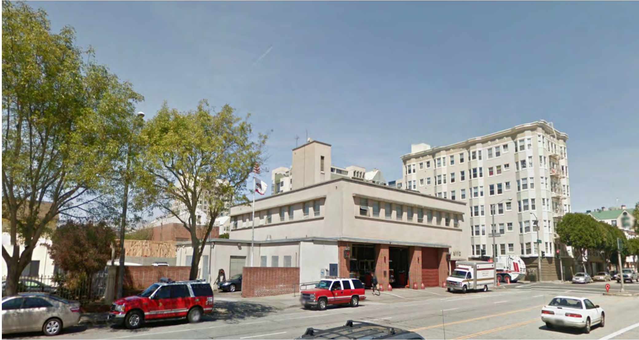
WEBSTER STREET - SOUTH & EAST FACADES
