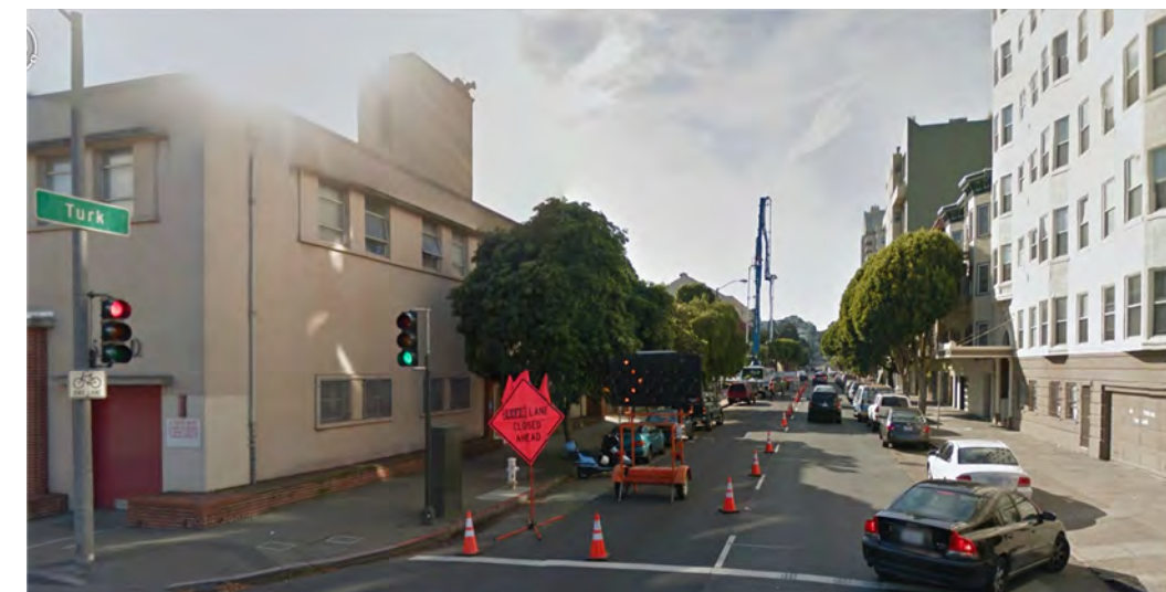
TURK STREET - NORTH FACADE
