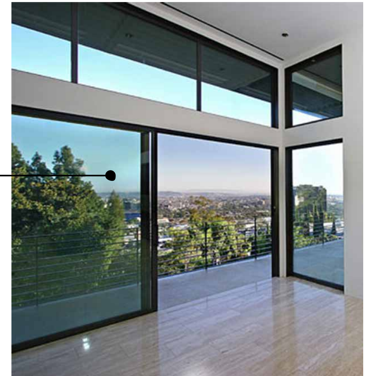
ANODIZED ALUMINUM MULTI-SLIDE WINDOW SYSTEM WESTERN WINDOW SYSTEMS SERIES 600
