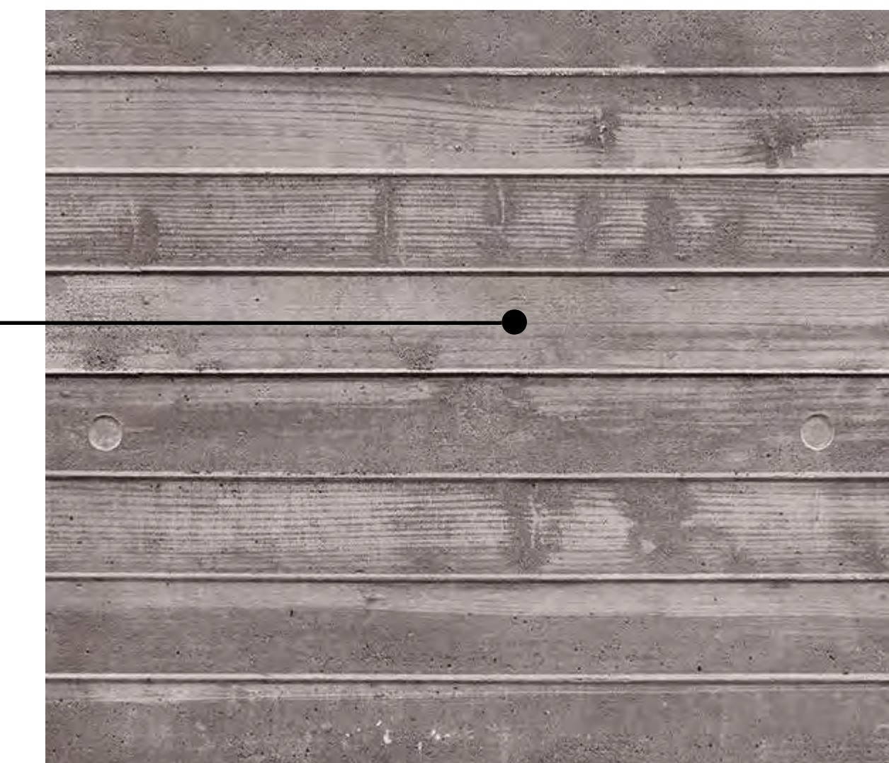
BOARD FORMED CONCRETE W/ SITE QUARRIED AGGREGATE
