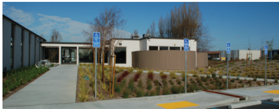
Main Building Entry
