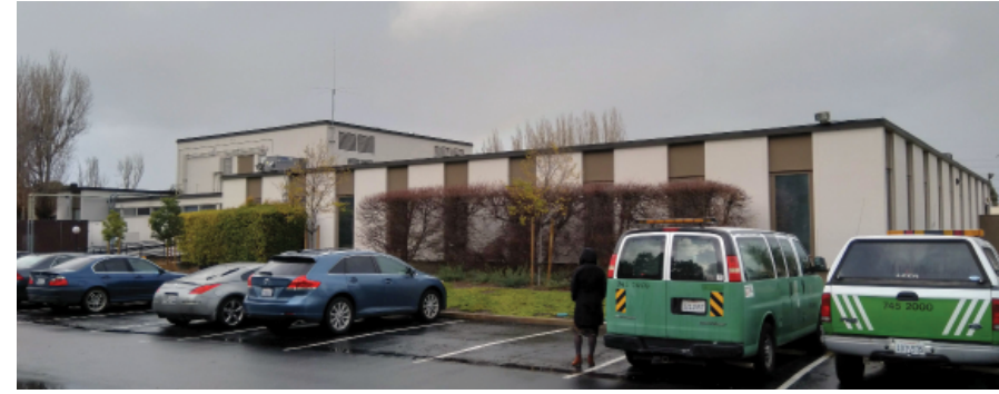
Existing Location for New Addition
