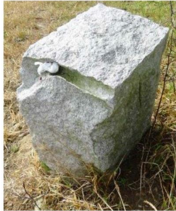
Before Treatment No. 71
