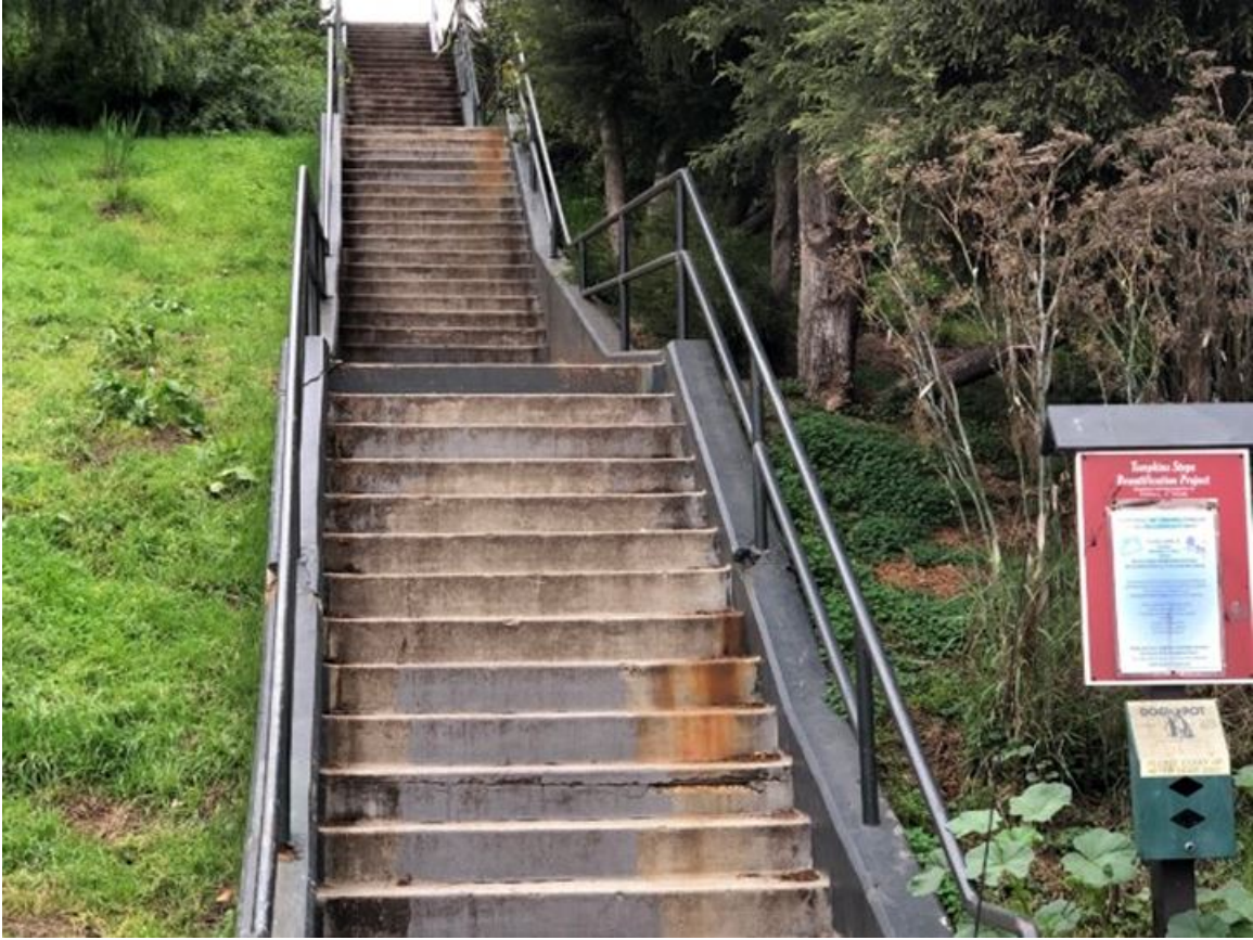
Tompkins Avenue stairs in 2017, prior to repairs and renovation
