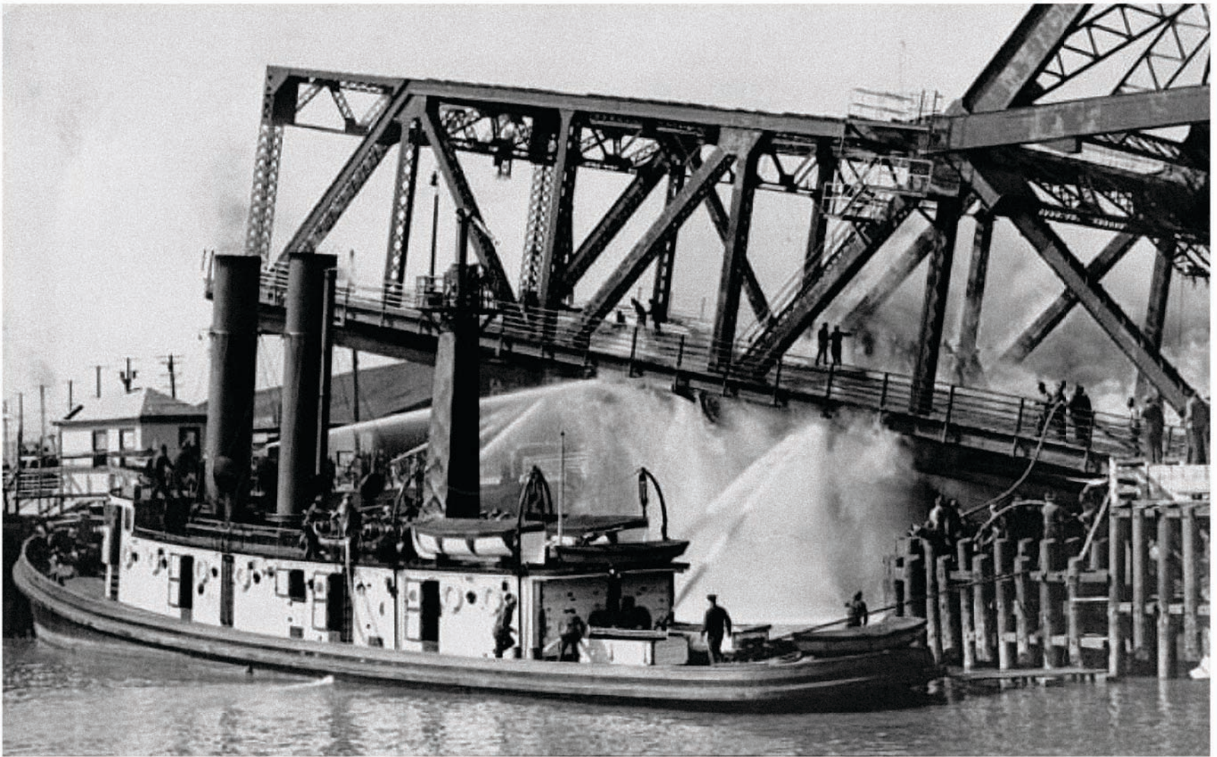
Fire fighters and fire boat extinguishing fire on Third street bridge San Francisco Public Library Historical Photograph Collection April 13th, 1933
