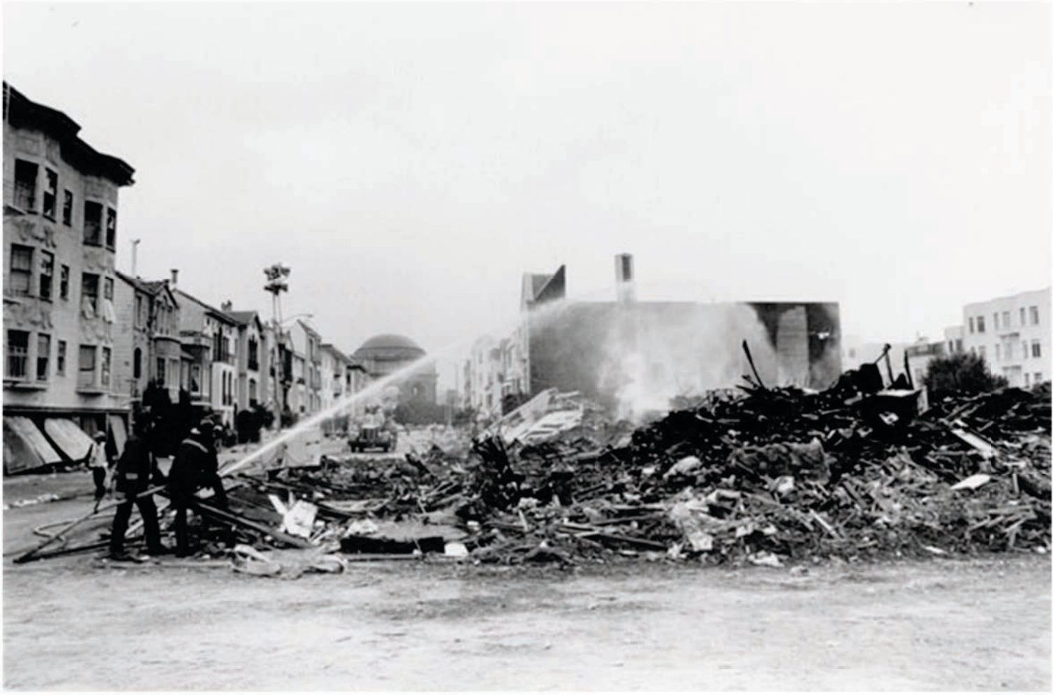
Firefighters putting out a fire in the Marina District caused by the Loma Prieta Earthquake Open SF History archives Oct 17, 1989, Loma Prieta
