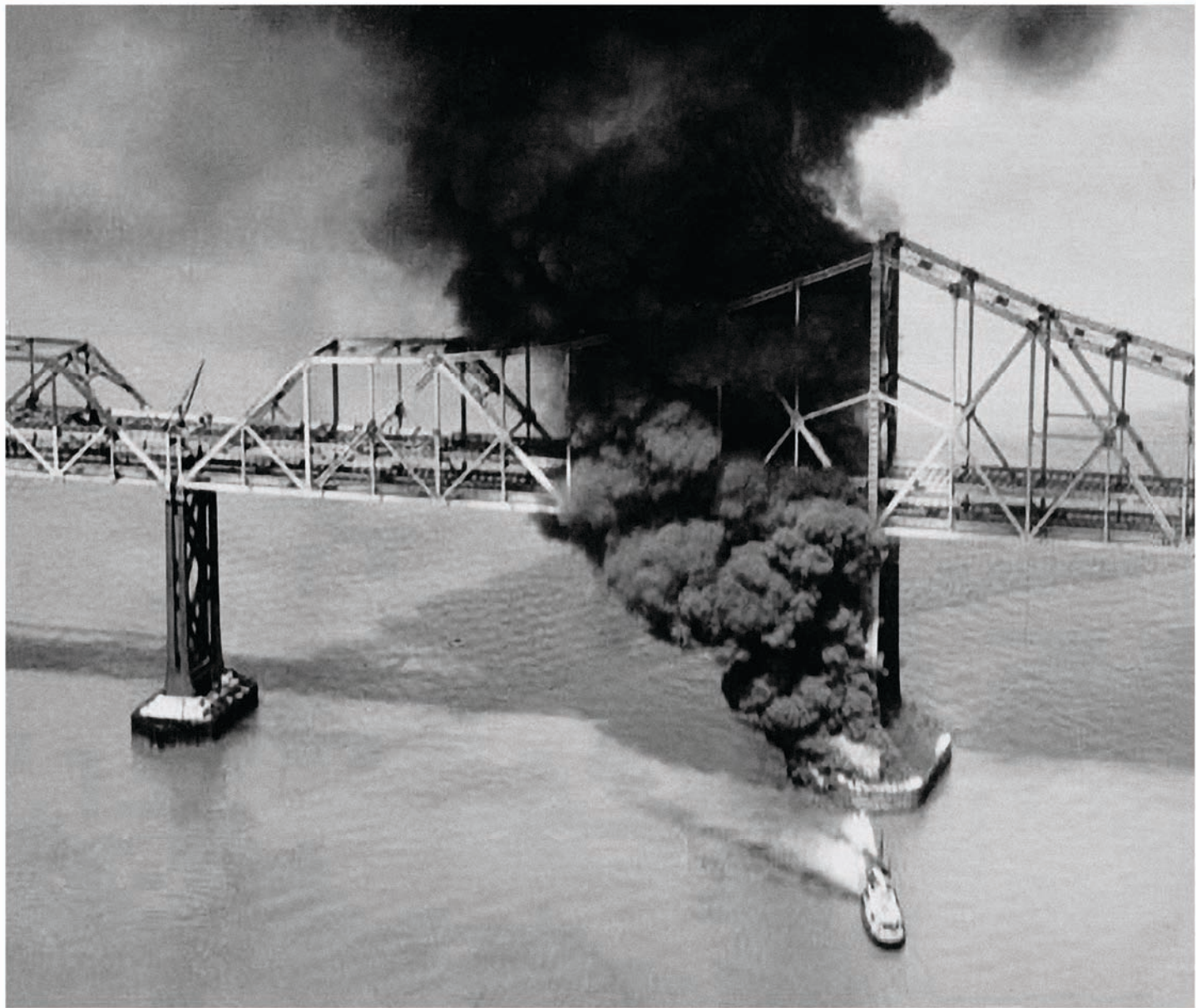
Fireboat fighting a fire on the cantilever section of the San Francisco-Oakland Bay Bridge San Francisco Public Library Historical Photograph Collection San Francisco, April 6th, 1936
