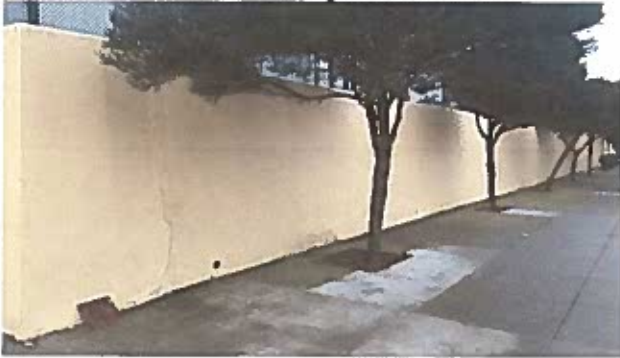
Morse Street looking west
