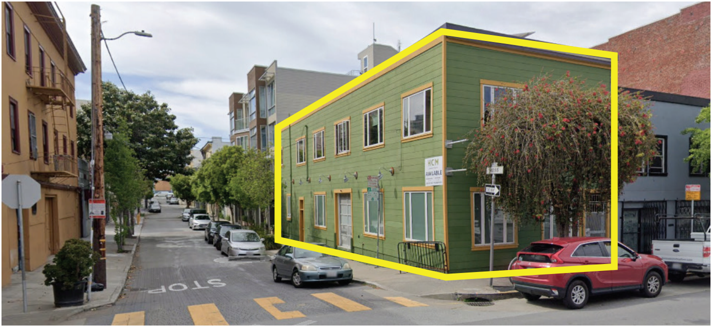
Existing view from Folsom Street
