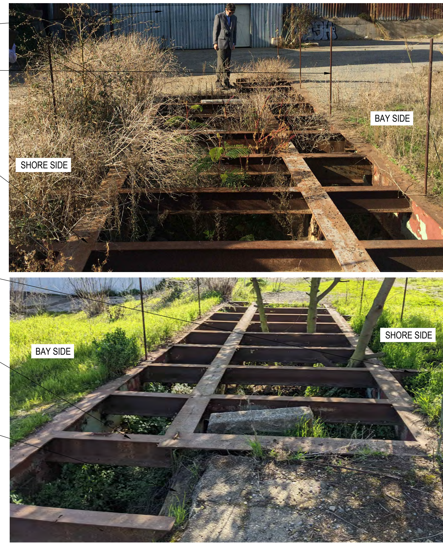
3 PHOTOS OF SALVAGED STRUCTURAL FRAME / GRILLAGE SCALE: 1" = 80'-0"
