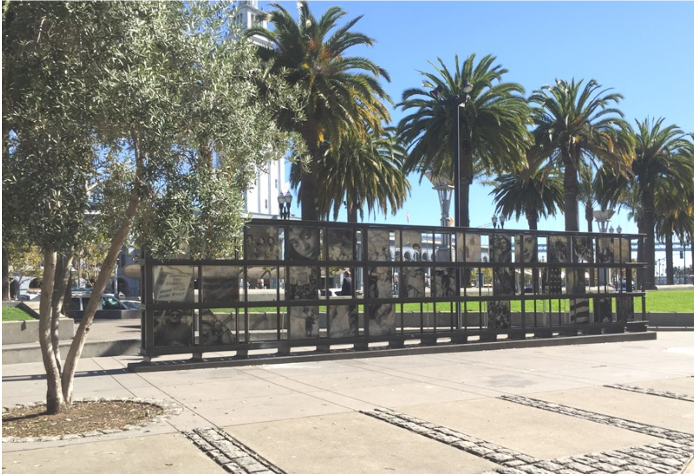
Abraham Lincoln Brigade National Monument, 2008 by Ann Chamberlin and Walter Hood (SFAC Accession No. 2008.3) Conservation Repair Design, 2016
