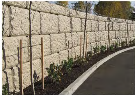
MSE RETAINING WALLS
