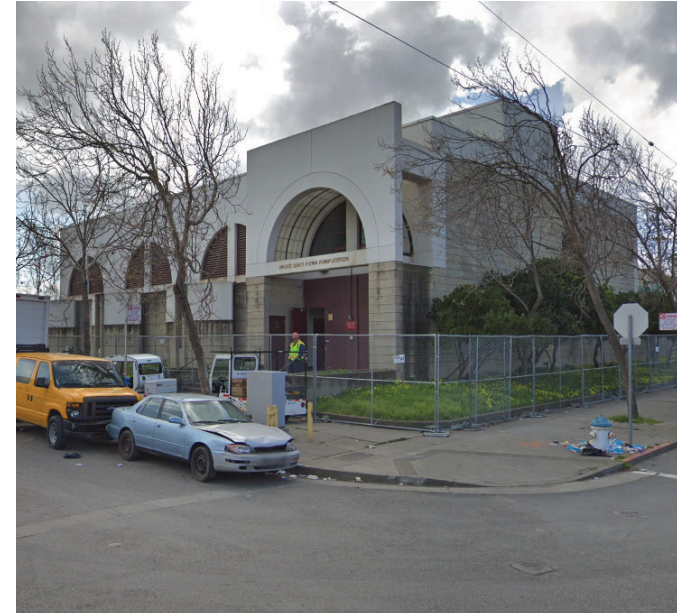
Bruce Flynn Pump Station
