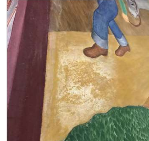
Figure 11: Detail of efflorescence on the Outdoor Life mural.
