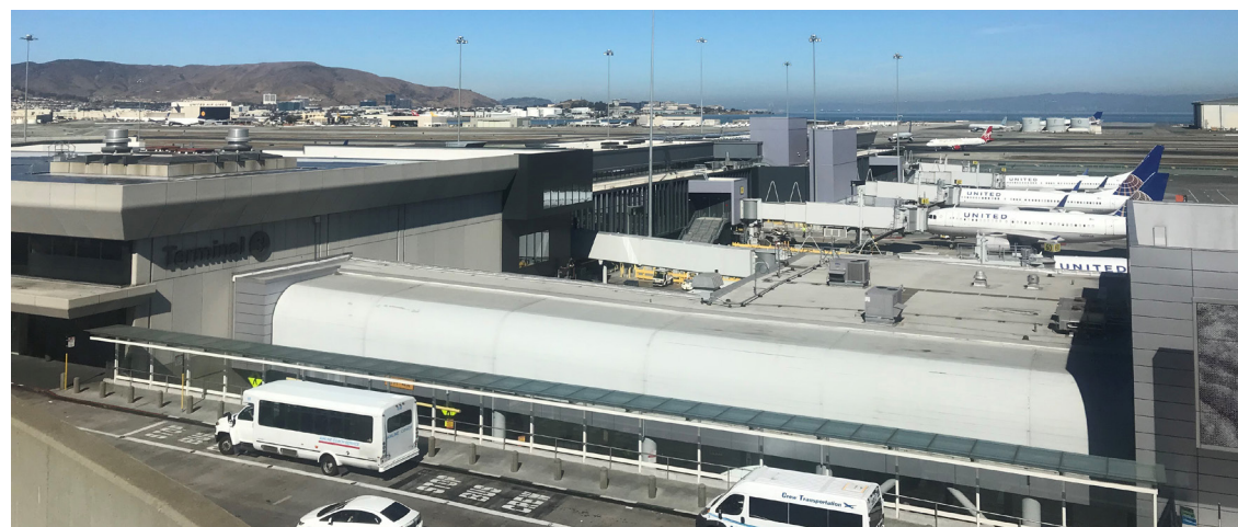
2. VIEW FROM PARKING GARAGE / AIR TRAIN PLATFORM
