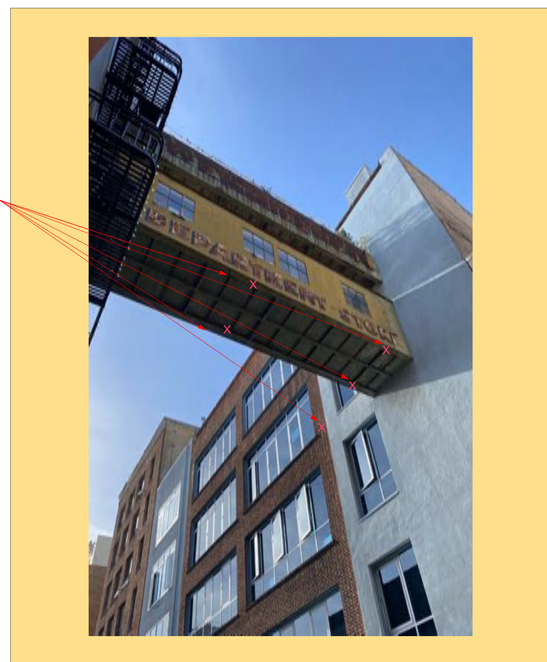
Image C: Anchor Points Attaching to Sky Bridge and Adjoining Buildings
