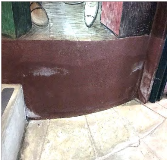
Figure 48: Detail of new efflorescence at the bottom of the stairs adjacent to the first-floor elevator door.
