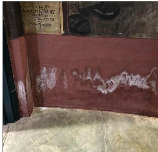
Figure 61: Detail of growing efflorescence at the bottom of the stairs on the stucco frame surrounding the Powell Street mural.
