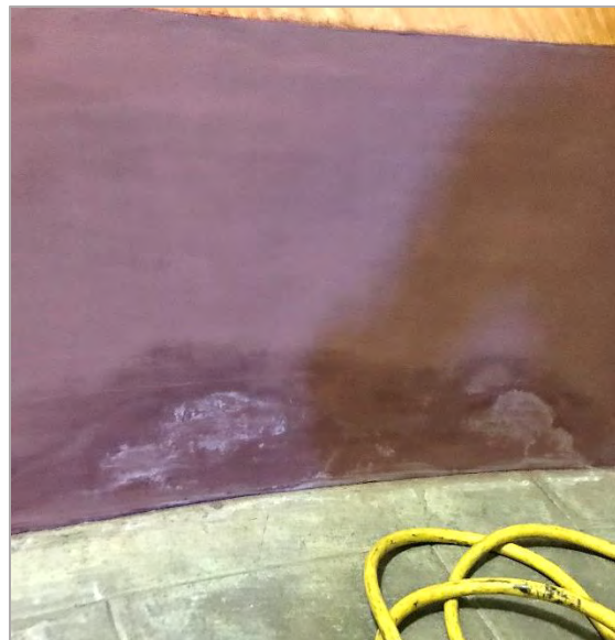
Figure 67: Growing efflorescence on the lower right side of the Outdoor Life mural.
