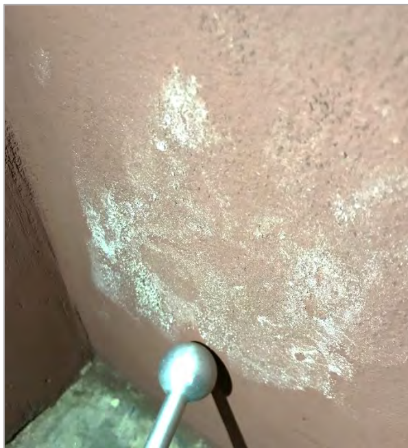
Figure 8: Detail of efflorescence on the same area.
