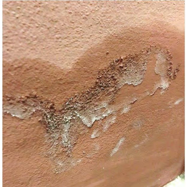
Figure 19: Detail of growing efflorescence at the bottom of the Powell Street mural's stucco frame. Notice wall still looks wet.
