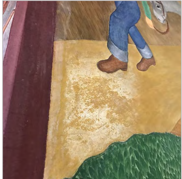
Figure 11: Detail of efflorescence on the Outdoor Life mural.
