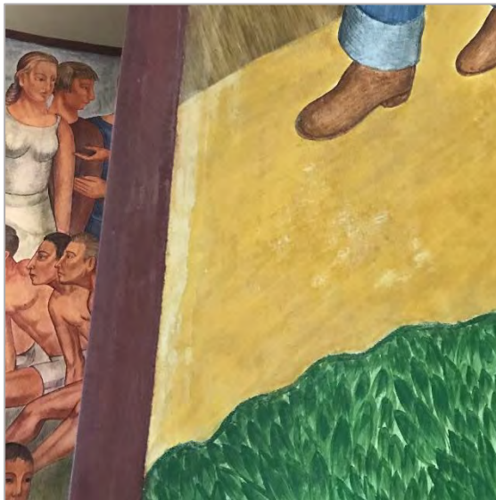
Figure 38: Detail of vertical stains, probably efflorescence, on the Outdoor Life mural. They appeared whiter and thicker in comparison to previous observations.
