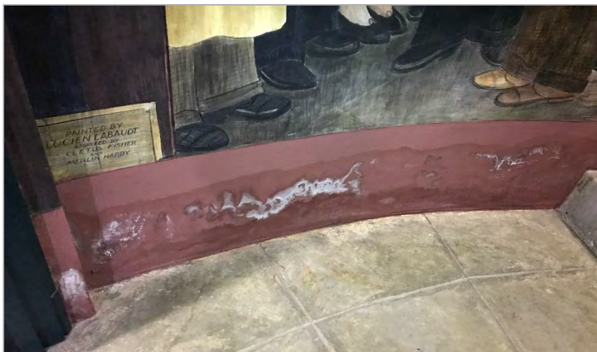
Figure 75: Detail of the central lower part of the Powell Street mural before water damage. Efflorescence this time are bigger and thicker than usual, which appeared right after the water leak.
