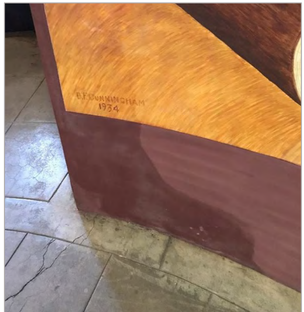
Figure 13: Detail of efflorescence on the Outdoor Life mural. Light accretions were emerging on the wall.
