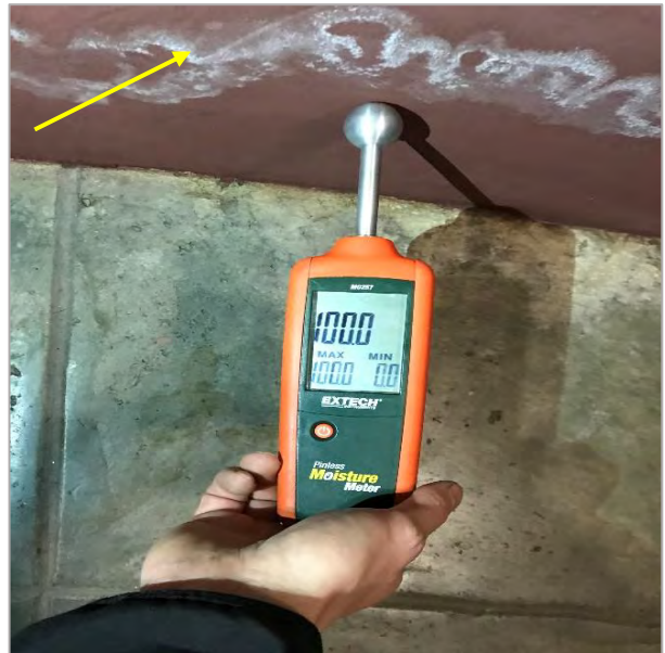
Figure 7: Yellow arrow shows heavy efflorescence on the stucco frame around the Powell Street mural.
