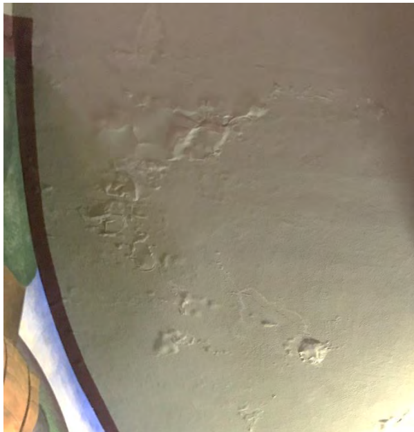
Figure 24: Detail of water damage on the second-floor ceiling.
