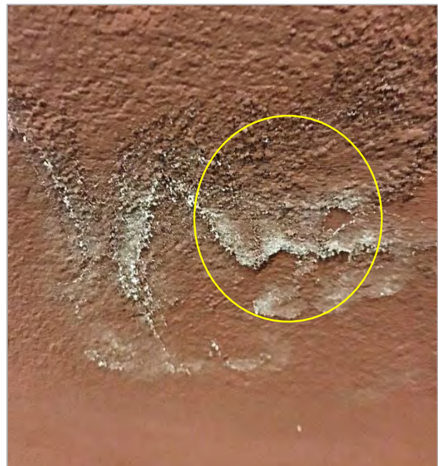
Figure 9: Detail of efflorescence on the same area. Yellow circle shows detail of the stucco paint being pulled away by efflorescence.
