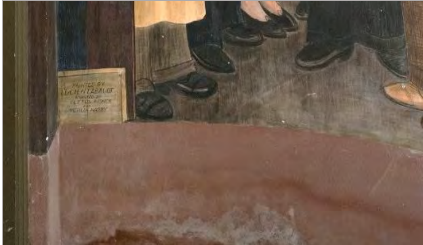
Figure 74: Detail of the central lower part of the Powell Street mural before water damage. Mild efflorescence in this area are common since this location always exhibits high percentage of water content in the winter.
