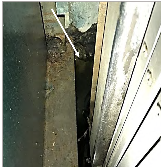
Figure 31: Detail of the accumulated water under the first-floor elevator. Arrow shows water level going up to the top of the elevator floor, which means that probably hundreds of gallons of water are currently contained in that area.
