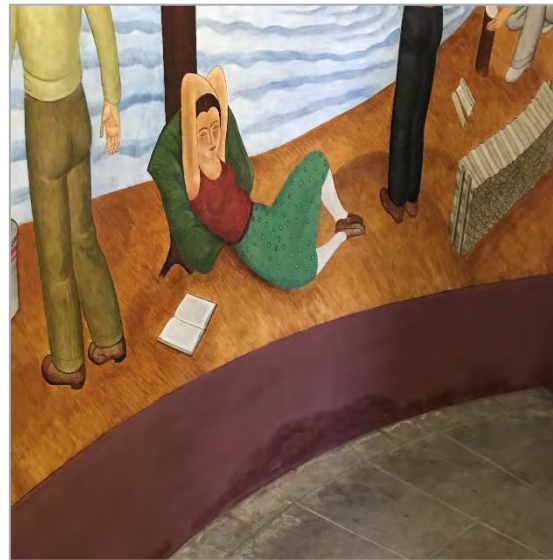
Figure 39: Efflorescence were starting to appear at the bottom of the frame of the Outdoor Life mural.
