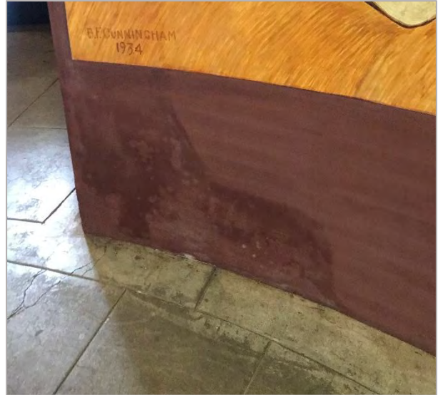
Figure 51: Location of observed efflorescence and other damages on the Outdoor Life mural.
