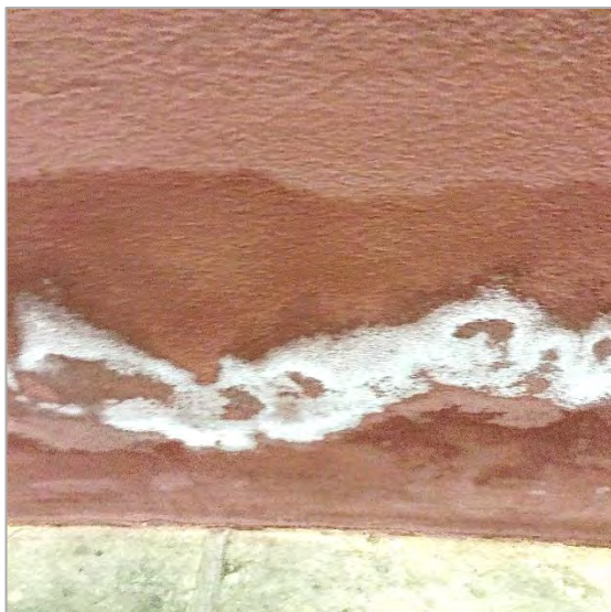
Figure 34: Detail of growing efflorescence at the bottom of the stairs on the frame surrounding the Powell Street mural.
