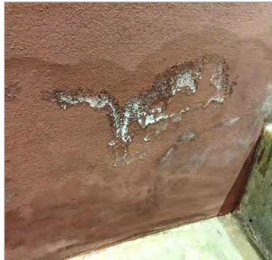
Figure 49: Detail of observed efflorescence and other damages on the Powell Street mural stucco frame.
