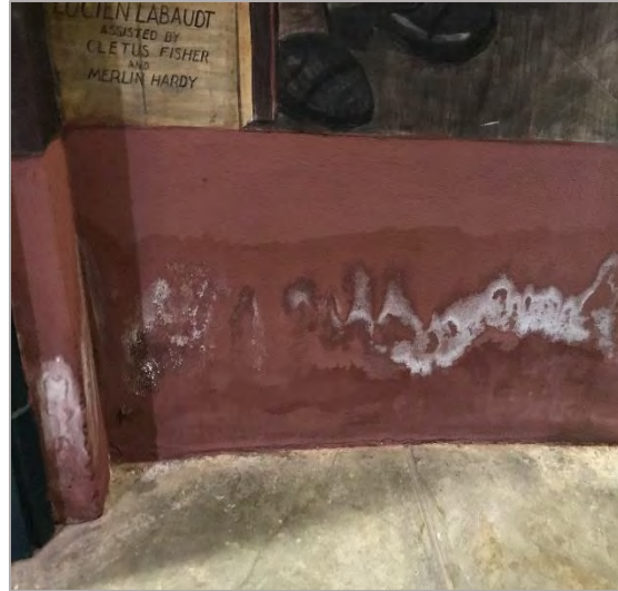
Figure 47: Detail of growing efflorescence at the bottom of the stairs on the stucco frame surrounding the Powell Street mural.
