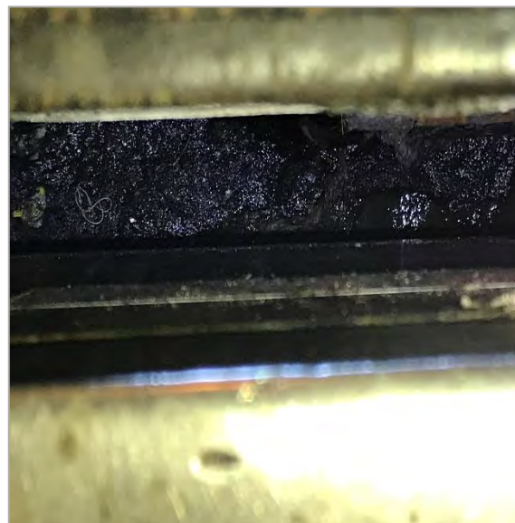
Figure 59: Water has been drained. Image shows bottom surface of the elevator. No water was observed.
