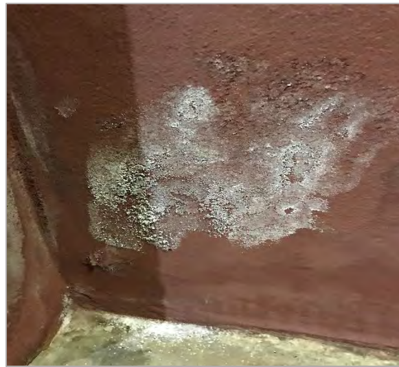
Figure 63: Detail of observed efflorescence and on the Powell Street mural stucco frame. Notice effloresce residues accumulated on the ground.
