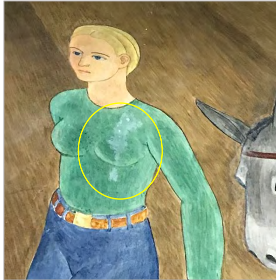
Figure 37: New white stain spotted, probably efflorescence, on the Outdoor Life mural.
