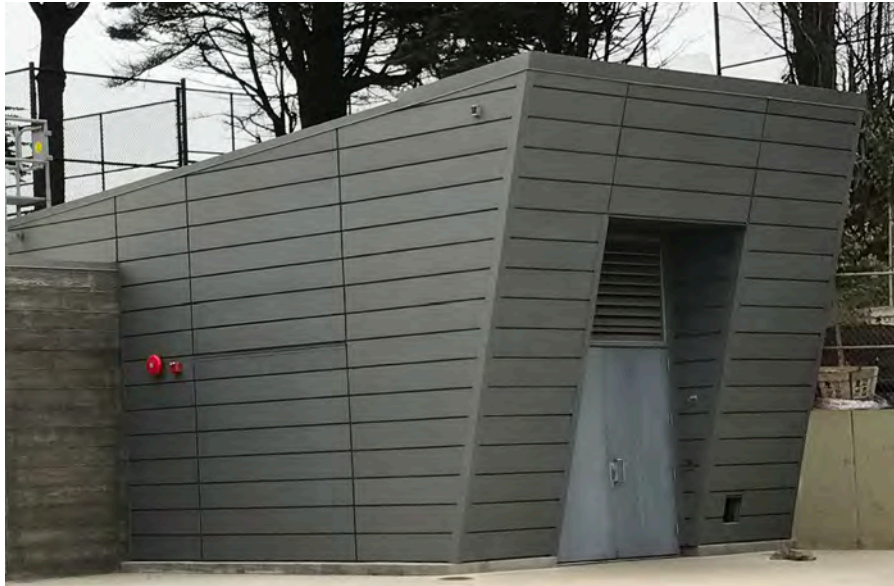
SFPUC WEST SUNSET PUMP STATION
