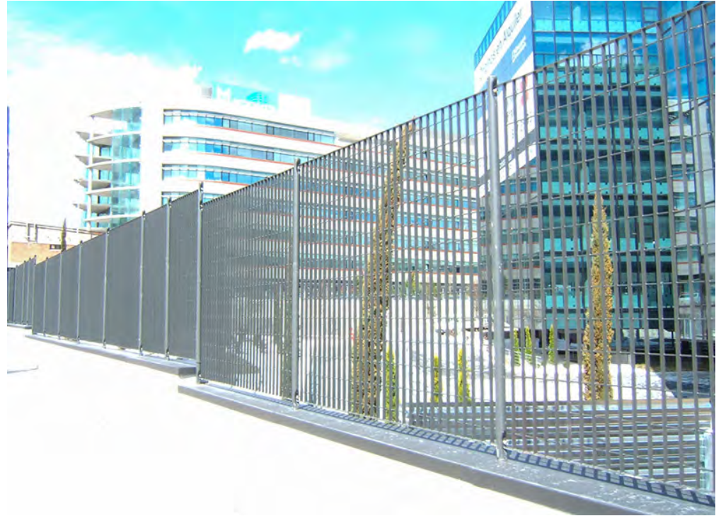
VERTICAL GRATING METAL FENCE
