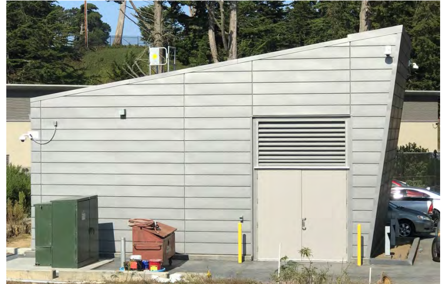
SFPUC LAKE MERCED PUMP STATION
