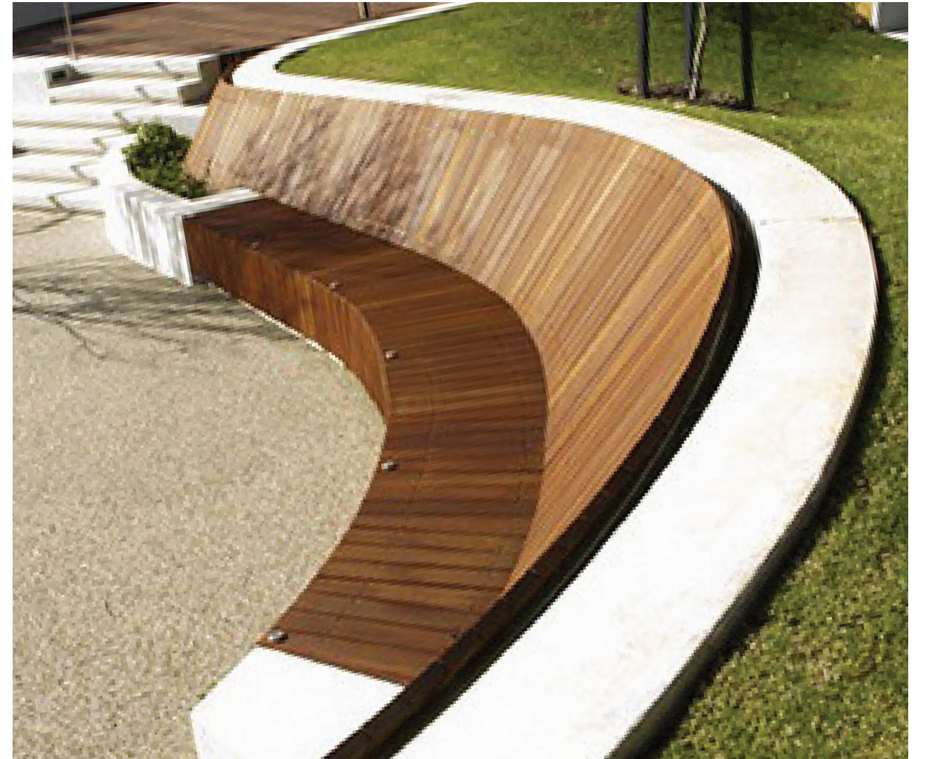
Wood seat and back integrated into retaining wall
