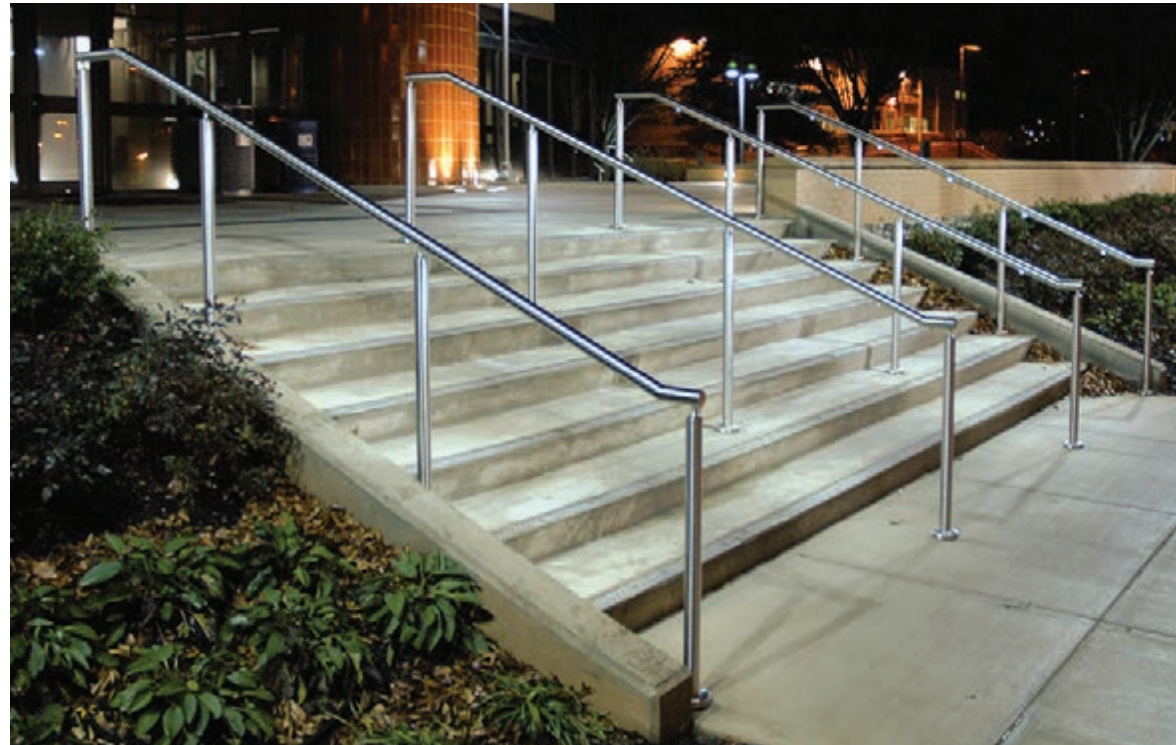
Galvanized lighted Handrail
