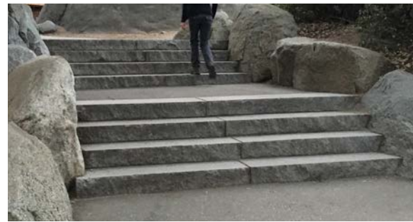
GRANITE STEPS W/ BOULDERS
