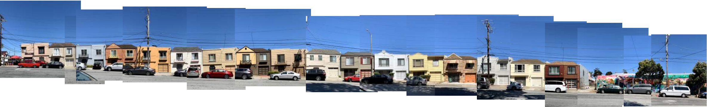
HAHN STREET LOOKING SOUTH EAST TOWARDS VISITACION VALLEY
