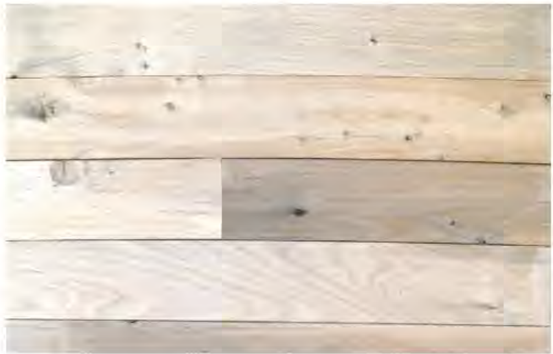
EXTERIOR - RESTORED FEATURES INTERIOR - NATURAL WOOD
