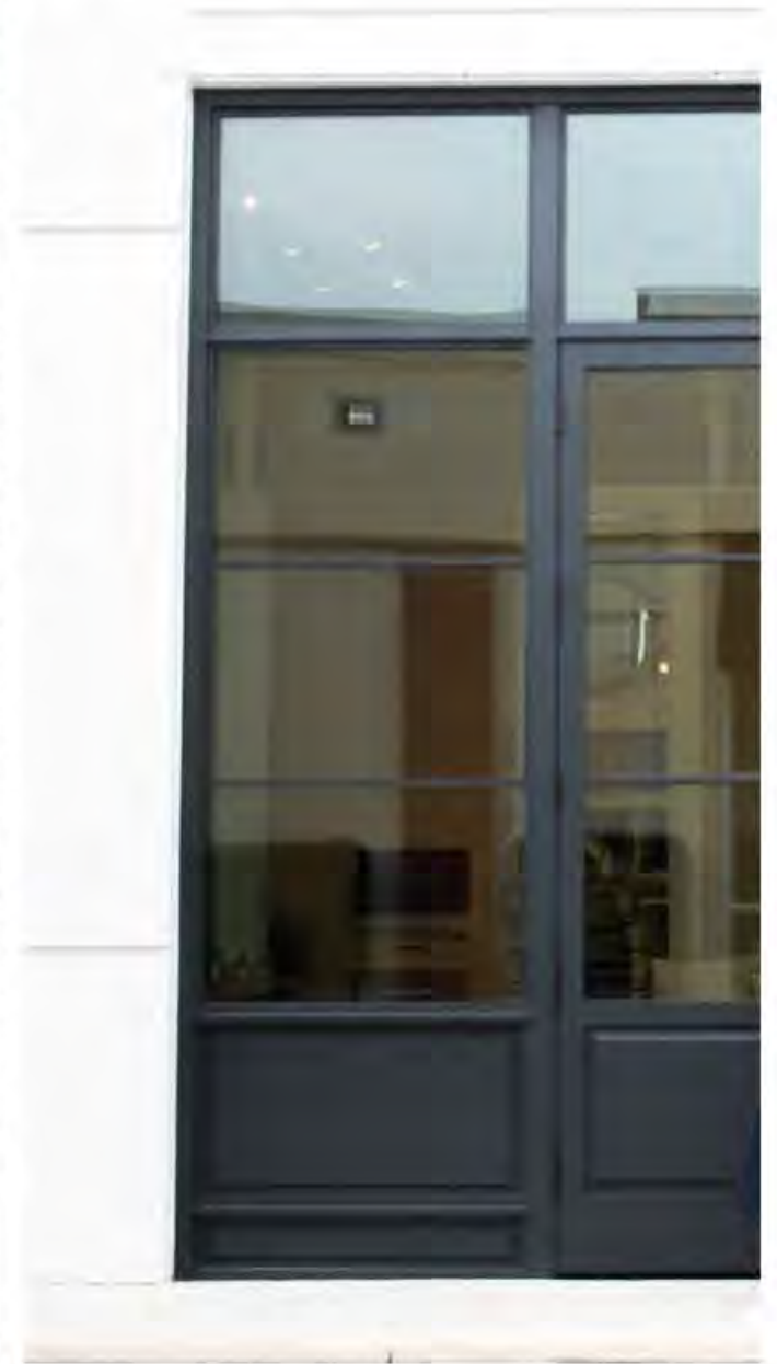
NEW OPENINGS - WOOD FRAME WITH EXTERIOR COATING
