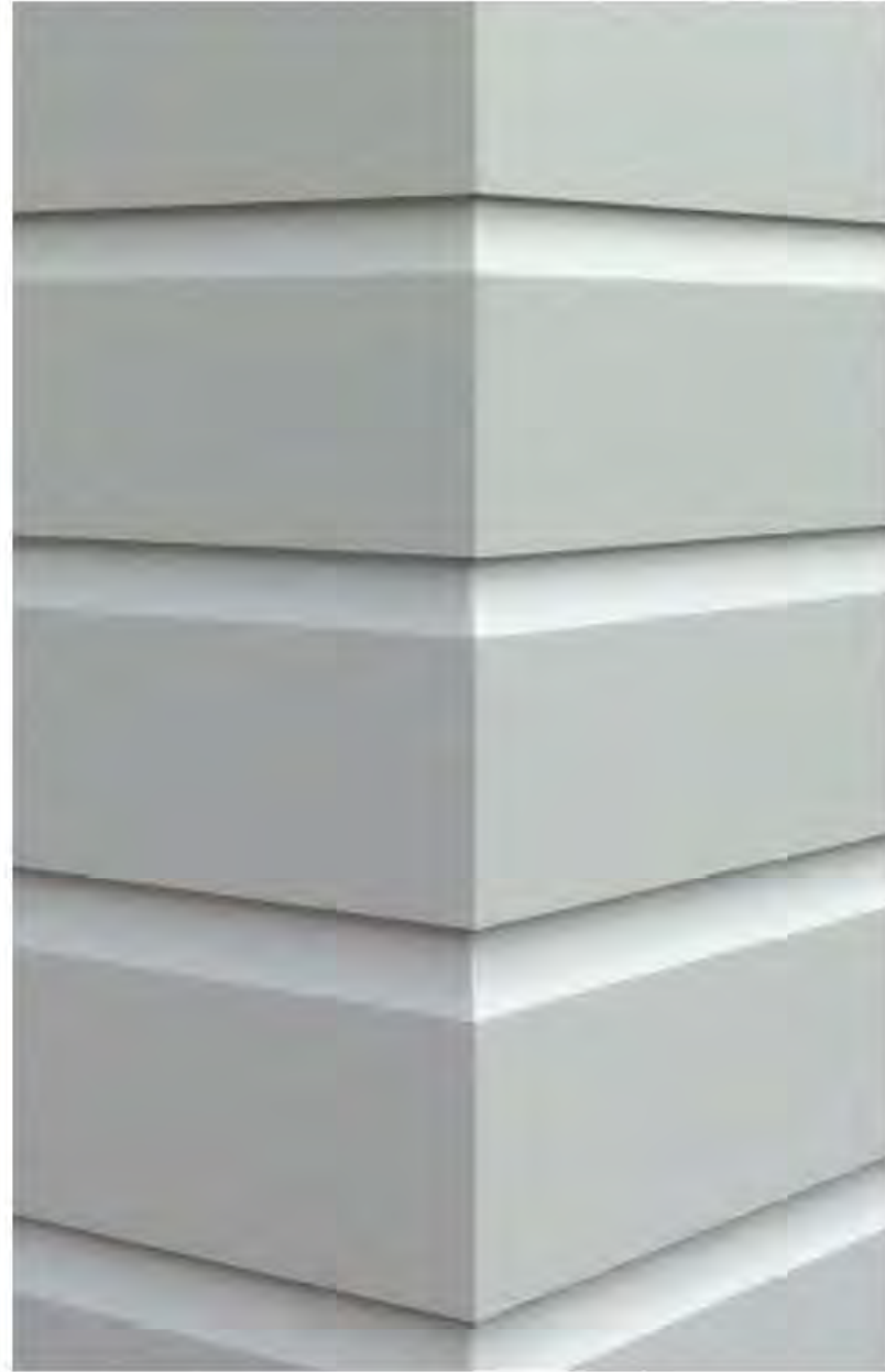
WALLS - RESTORED WOOD SIDING
