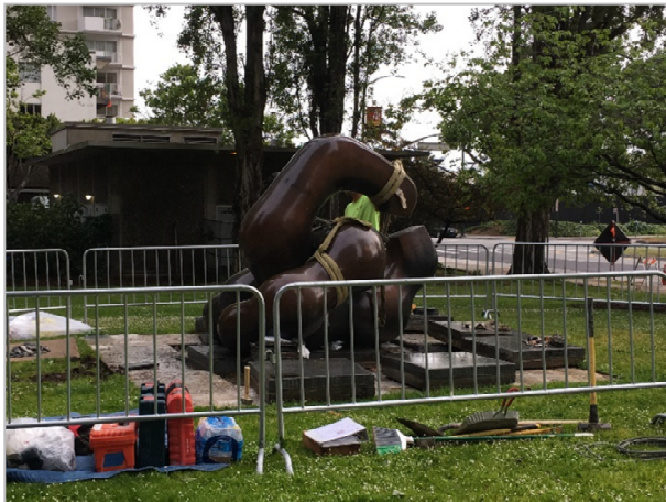
Image 5: Sculpture being removed from Sue Biermann Park via crane.
