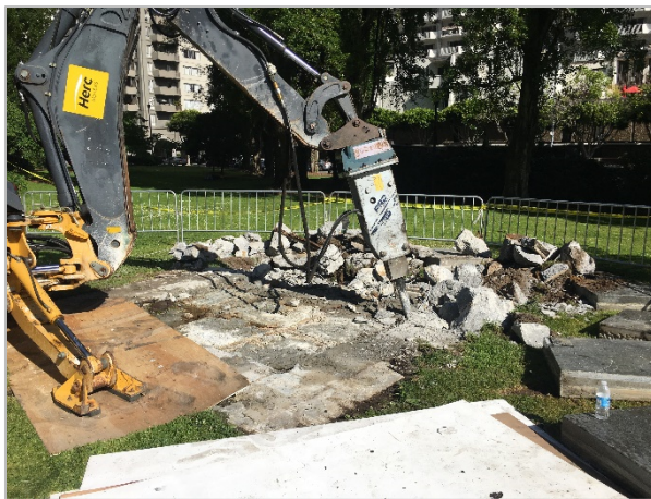
Image 7: Demolition of the concrete base after removal of the sculpture.
