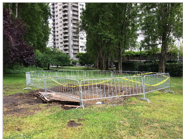
Image 8: Overall view of site after removal and demolition of base.
