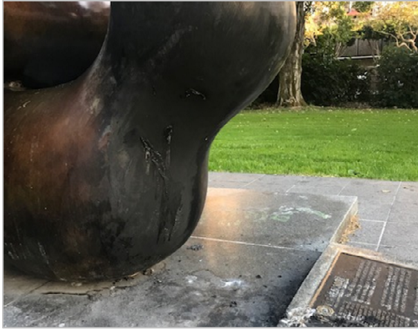
Image 1: Detail image of damaged patina from fire.
