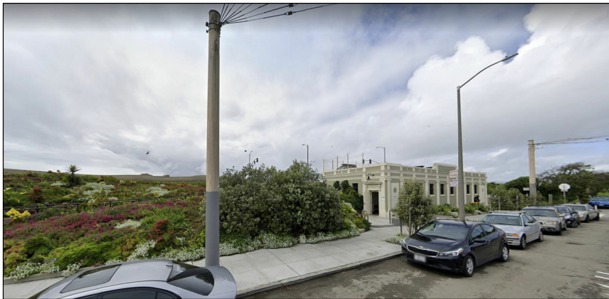
VIEW 1: CORNER OF JUDAH PUBLIC CONVENIENCE STATION
