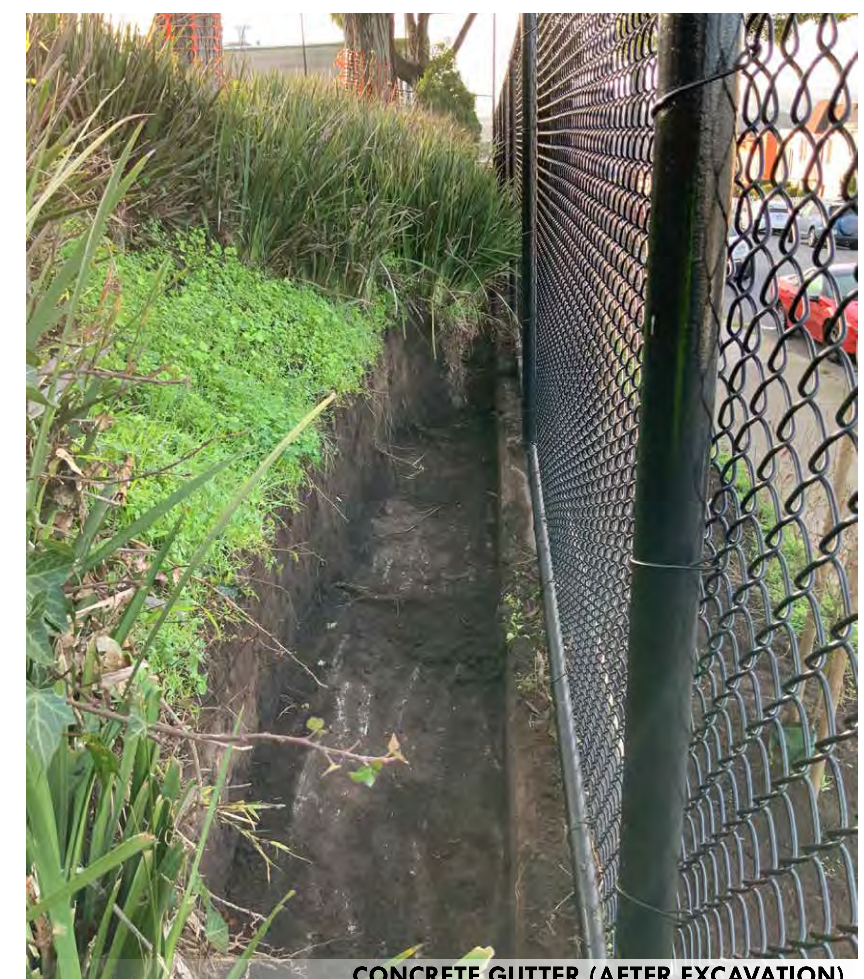
CONCRETE GUTTER (AFTER EXCAVATION)
