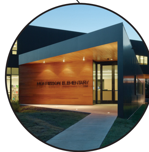
WARM ENTRY WITH T&G WOOD WALL AND SOFFIT
