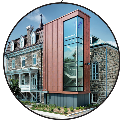
METAL PANEL CLAD CIRCULATION ADDITION
