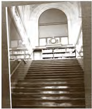
Original stairs and window
