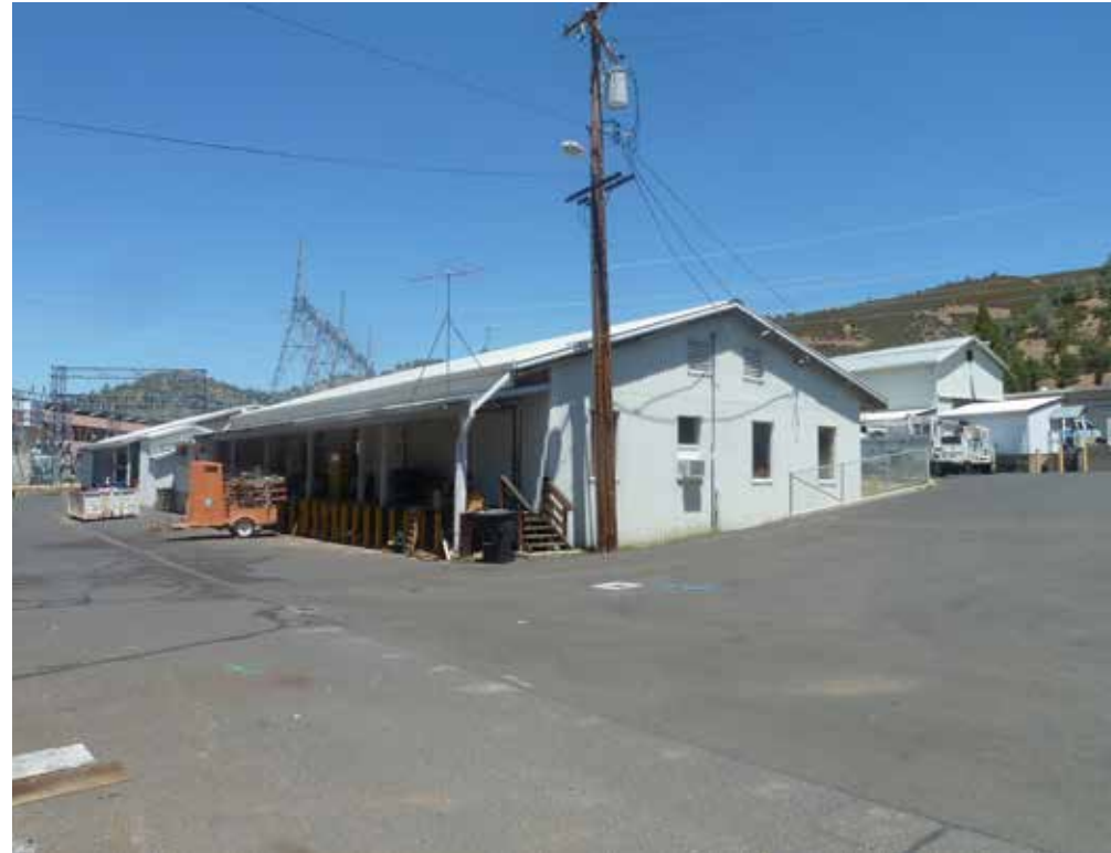
Field Office/Tool Room/Plumbing Shop
