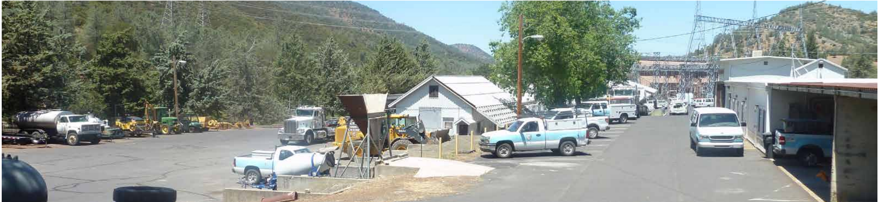
Materials Bin and, Old Paint Shop, and the proposed site of Building 76
