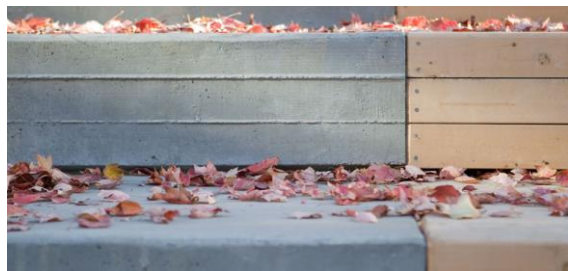
Board Form Concrete and Wood Steps
