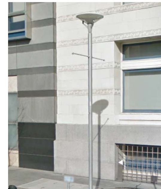
Oak Street Pole Light (Existing Light at Conservatory)
