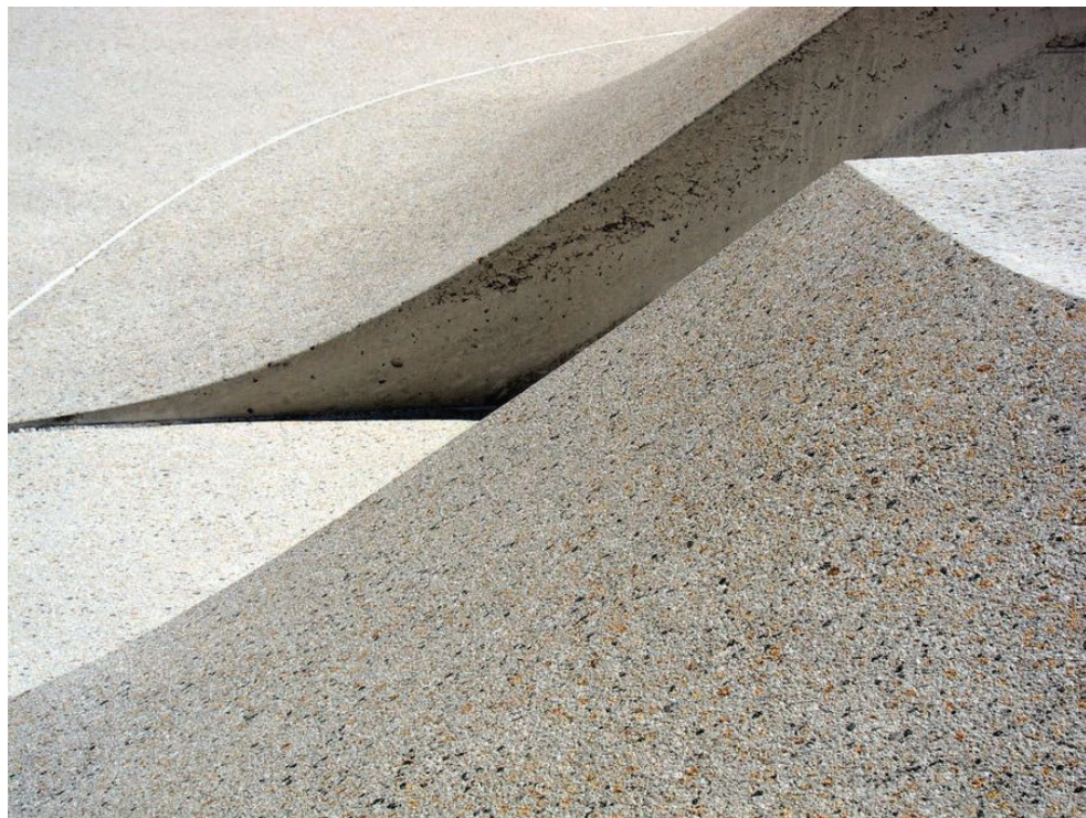
CAST IN PLACE CONCRETE
