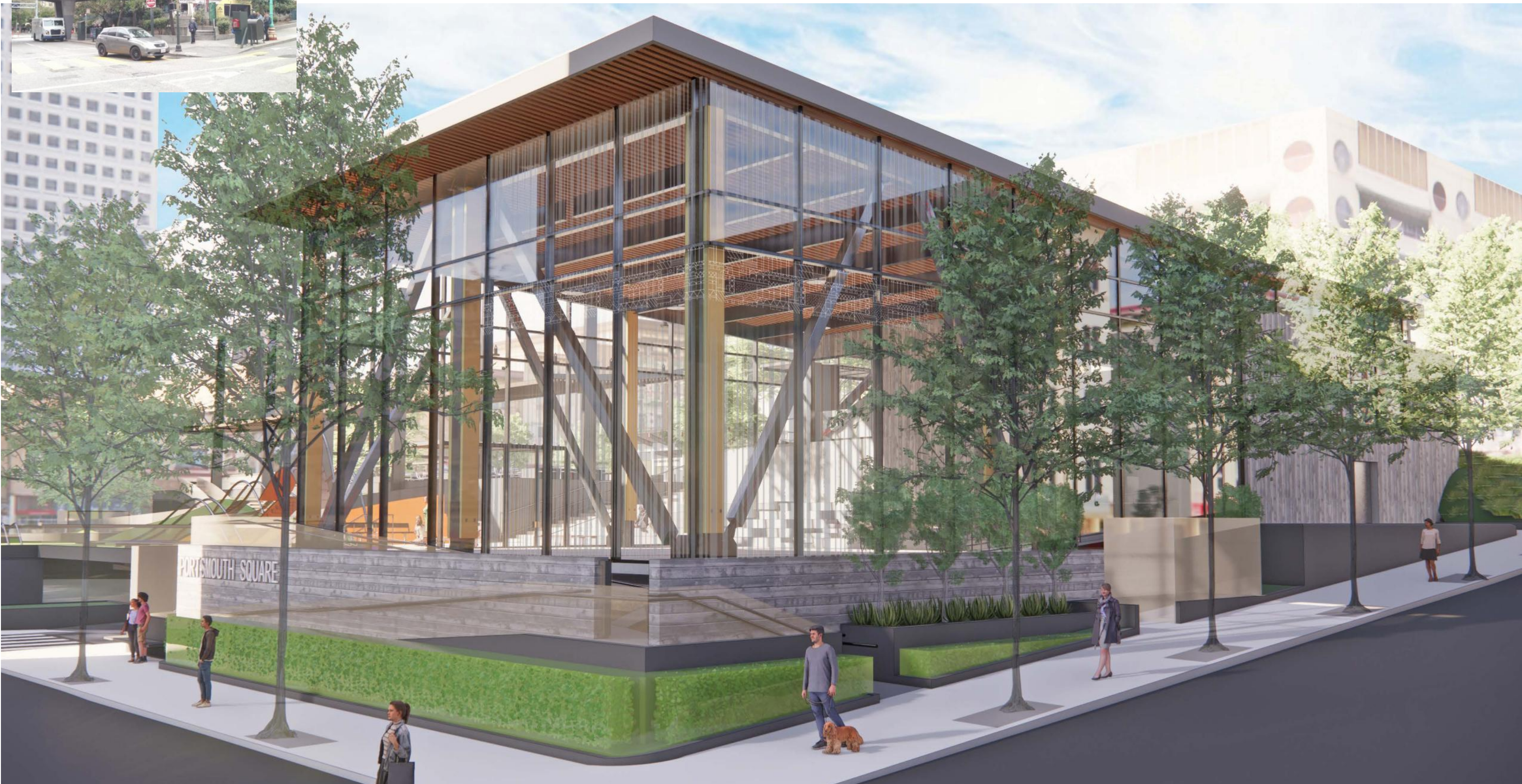
EXTERIOR FROM WITHIN PORTSMOUTH SQUARE
