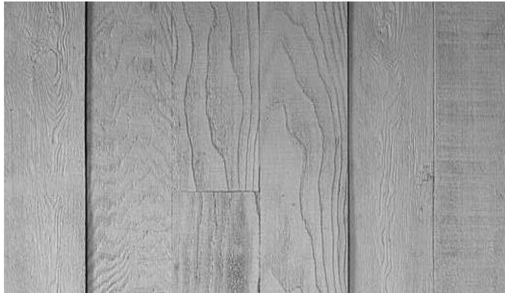
BOARD FORMED CONCRETE WALLS- 2/240 BALI FORM BY RECKLI/SLNDERWALL
