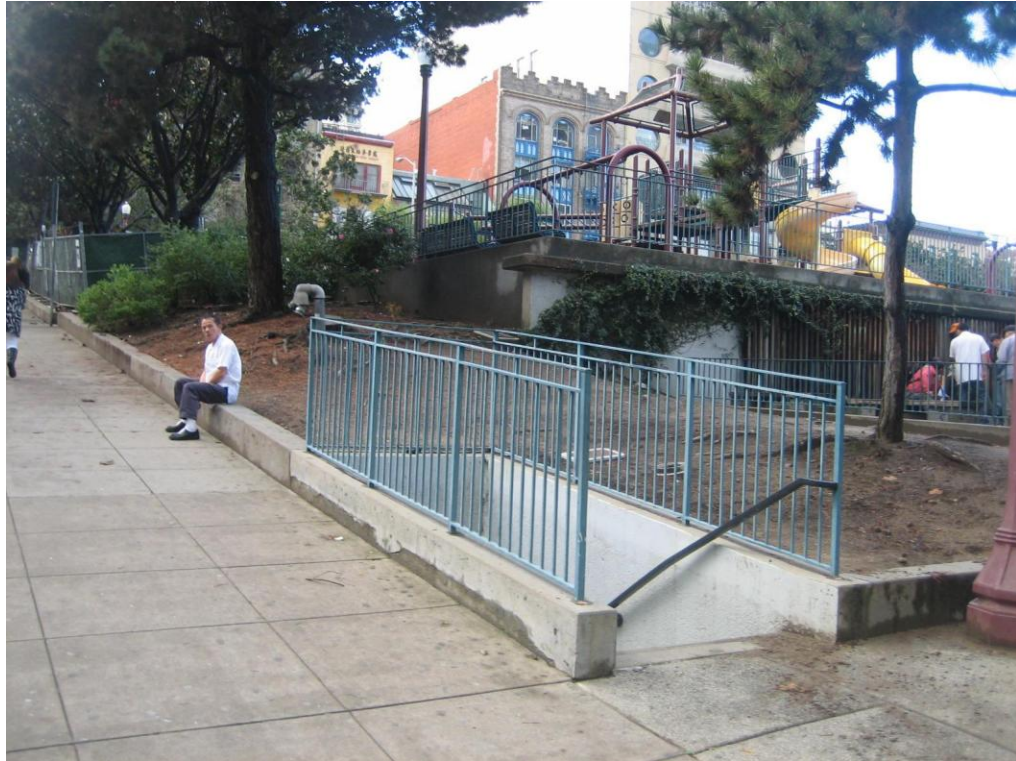
STAIRS #1 ON CLAY STREET
