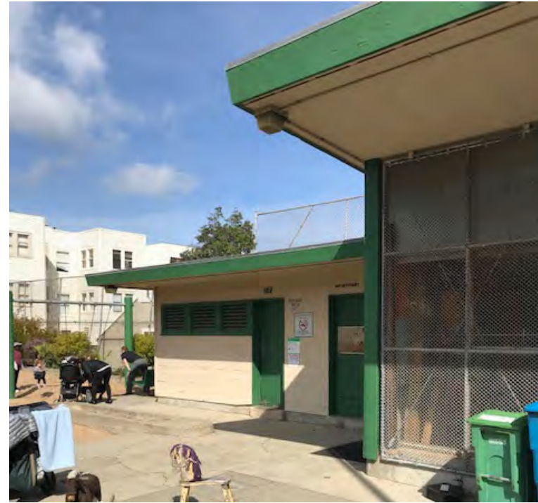
Richmond Playground Clubhouse Looking NW
