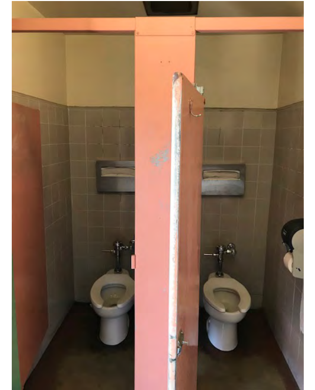
(E) Women's restroom interior
