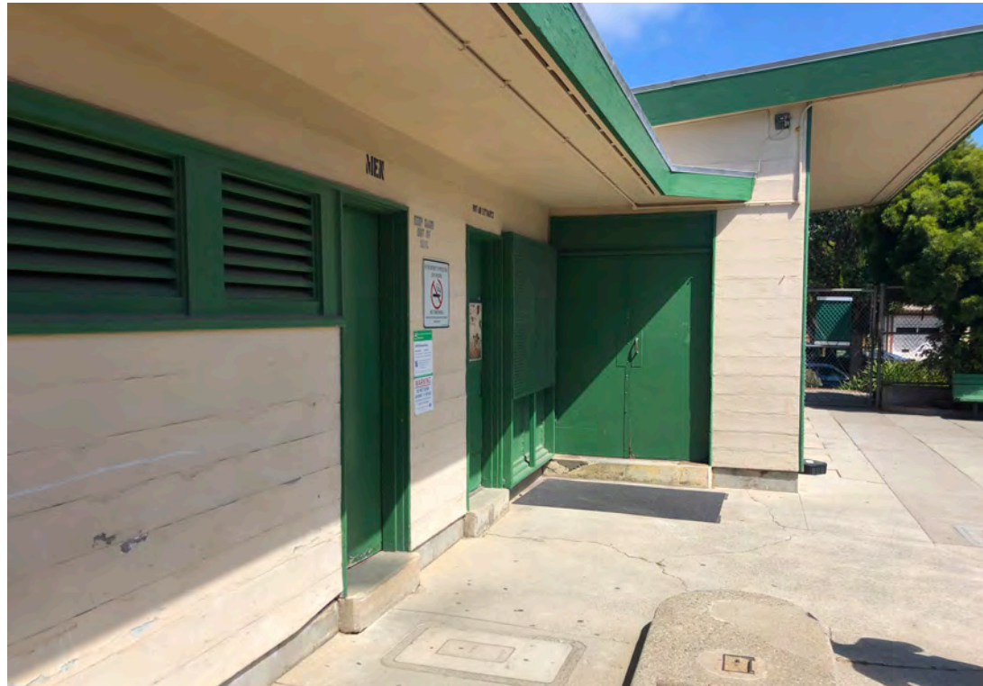
(E) Men's restroom exterior
