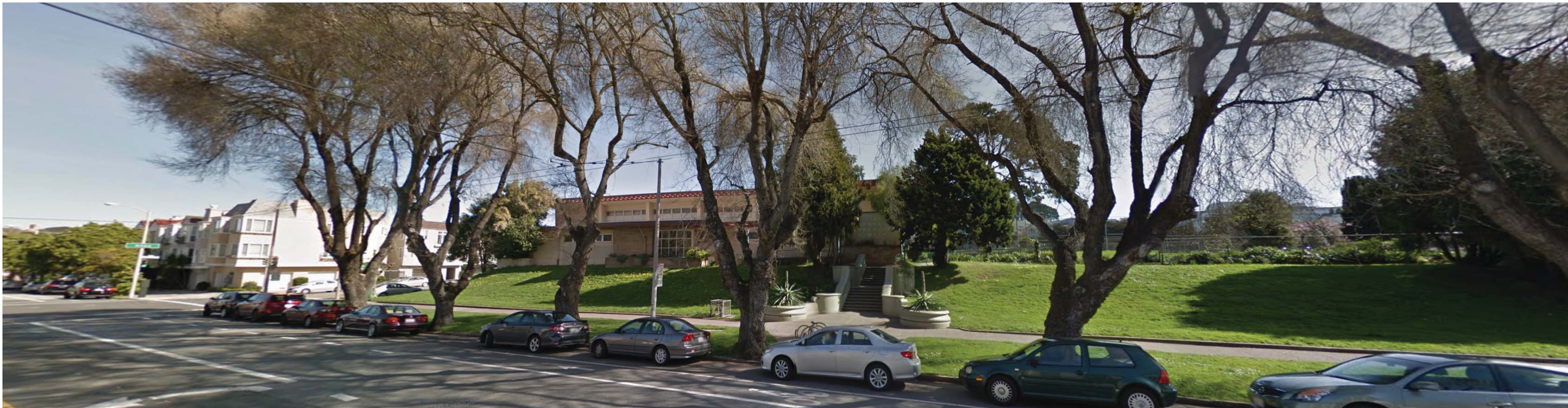
ARGUELLO BOULEVARD - SOUTHWEST VIEW - POOL BUILDING MAIN ENTRY
