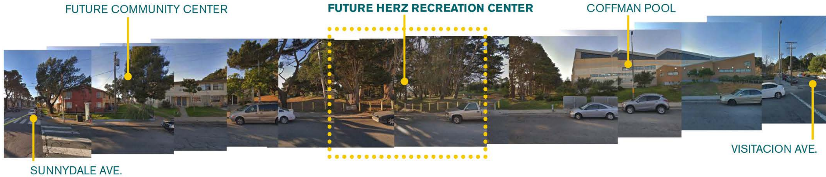
HAHN STREET LOOKING NORTH WEST TOWARDS MCLAREN PARK
