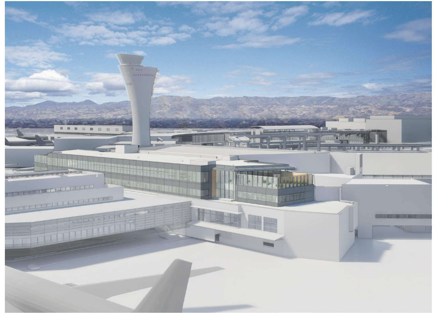
Phase 2 Aerial View
