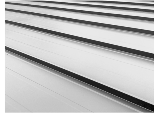
METAL STANDING SEAM ROOFING
