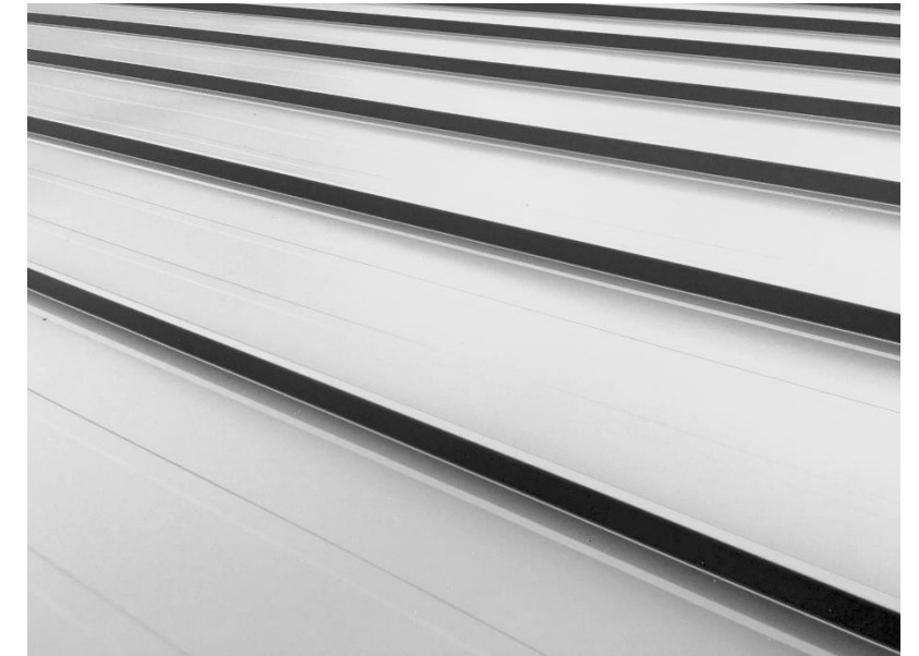
METAL STANDING SEAM ROOFING
