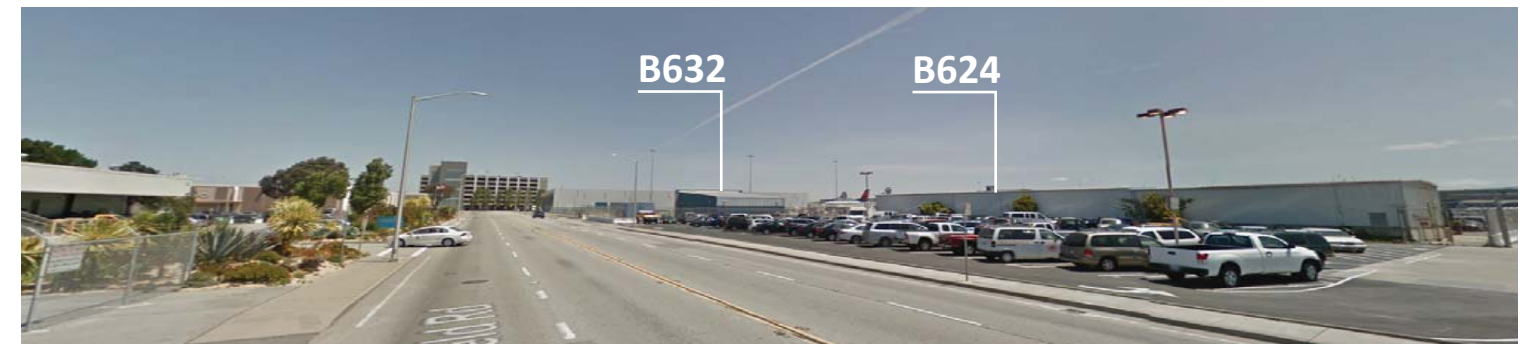
Looking at Existing B624 towards West Field Road
