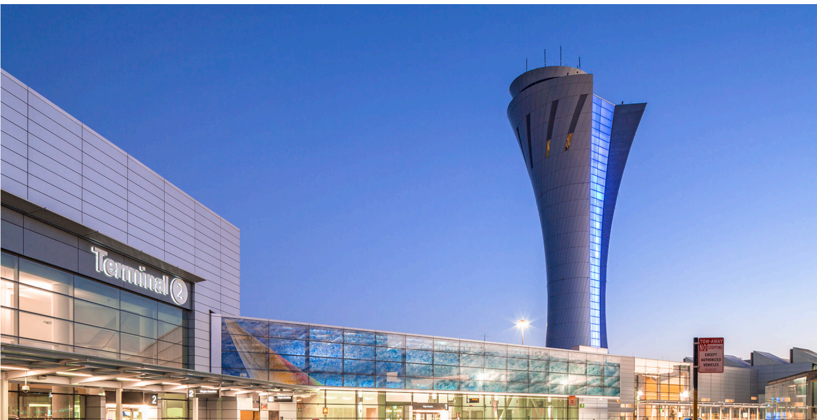
AIR TRAFFIC CONTROL TOWER
