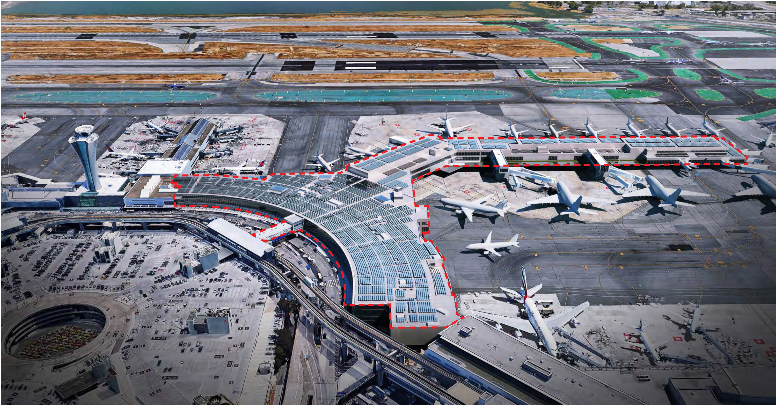
San Francisco International Airport Terminal 1 Renovation
