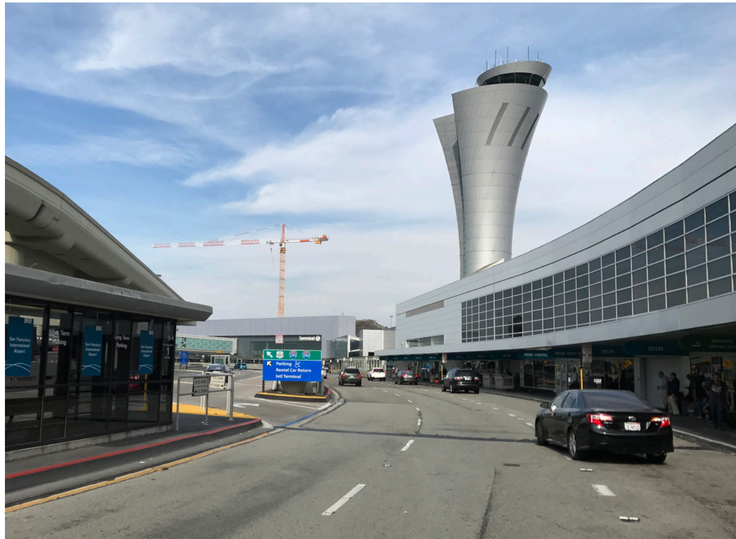
Curbside View after Tower Demolition
