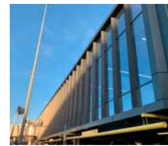
VERTICAL MULLIONS (BOARDING AREA E)
