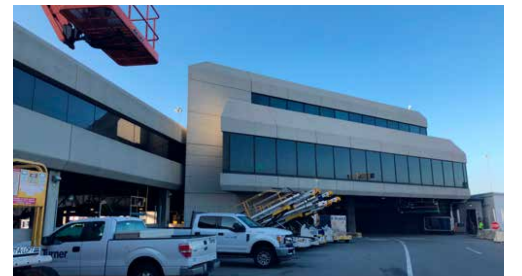
C. EXISTING FACADE
