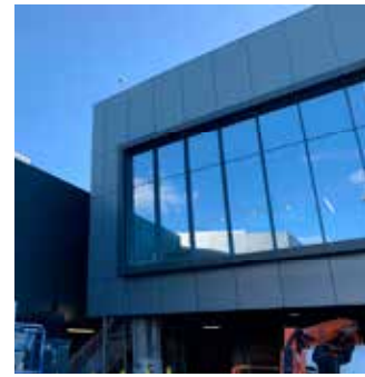
METAL BROW SURROUND (TERMINAL 3 EAST)
