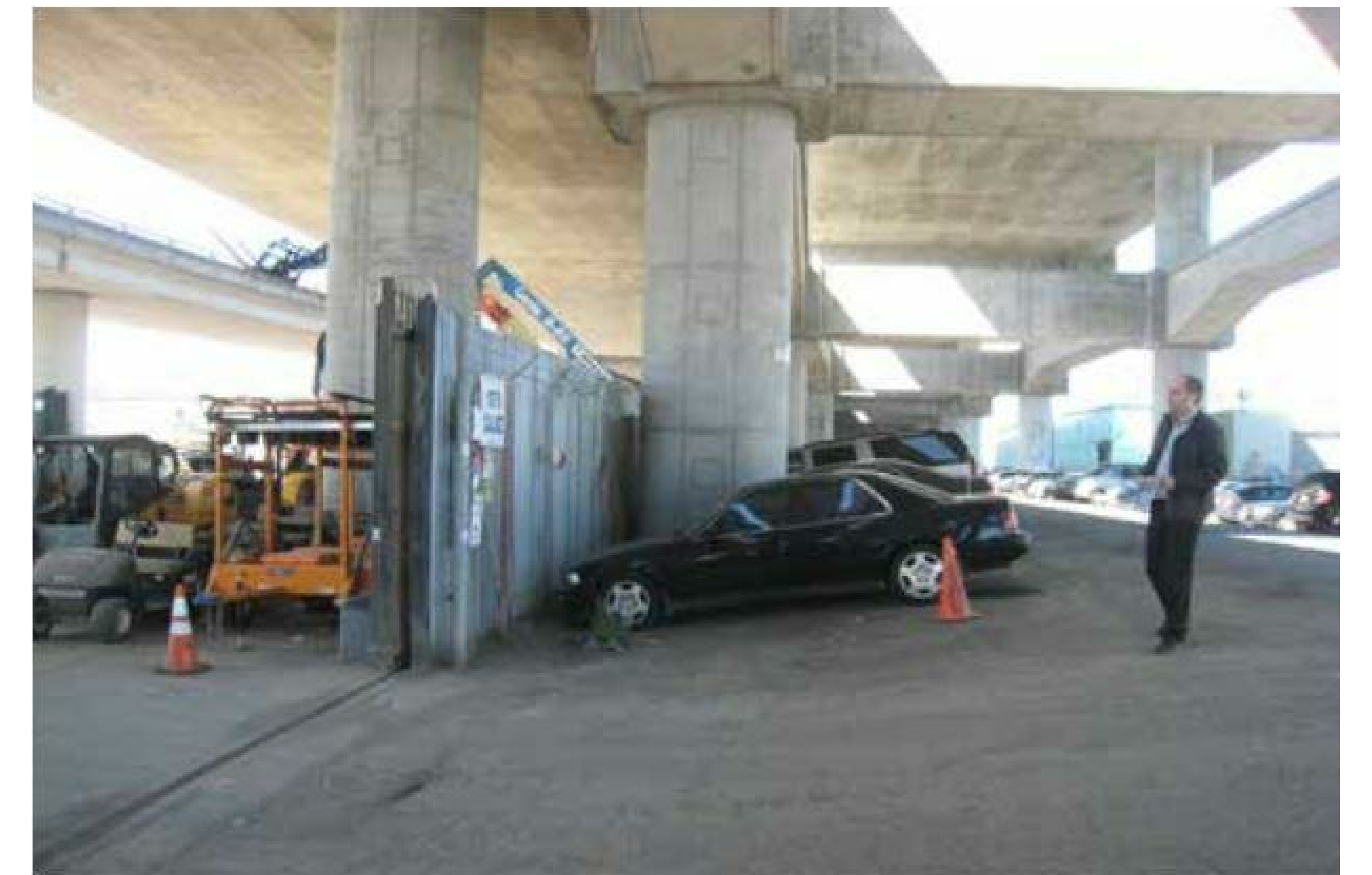
6 VIEW OF SLOPE FROM SELBY STREET INTO PROJECT SITE
