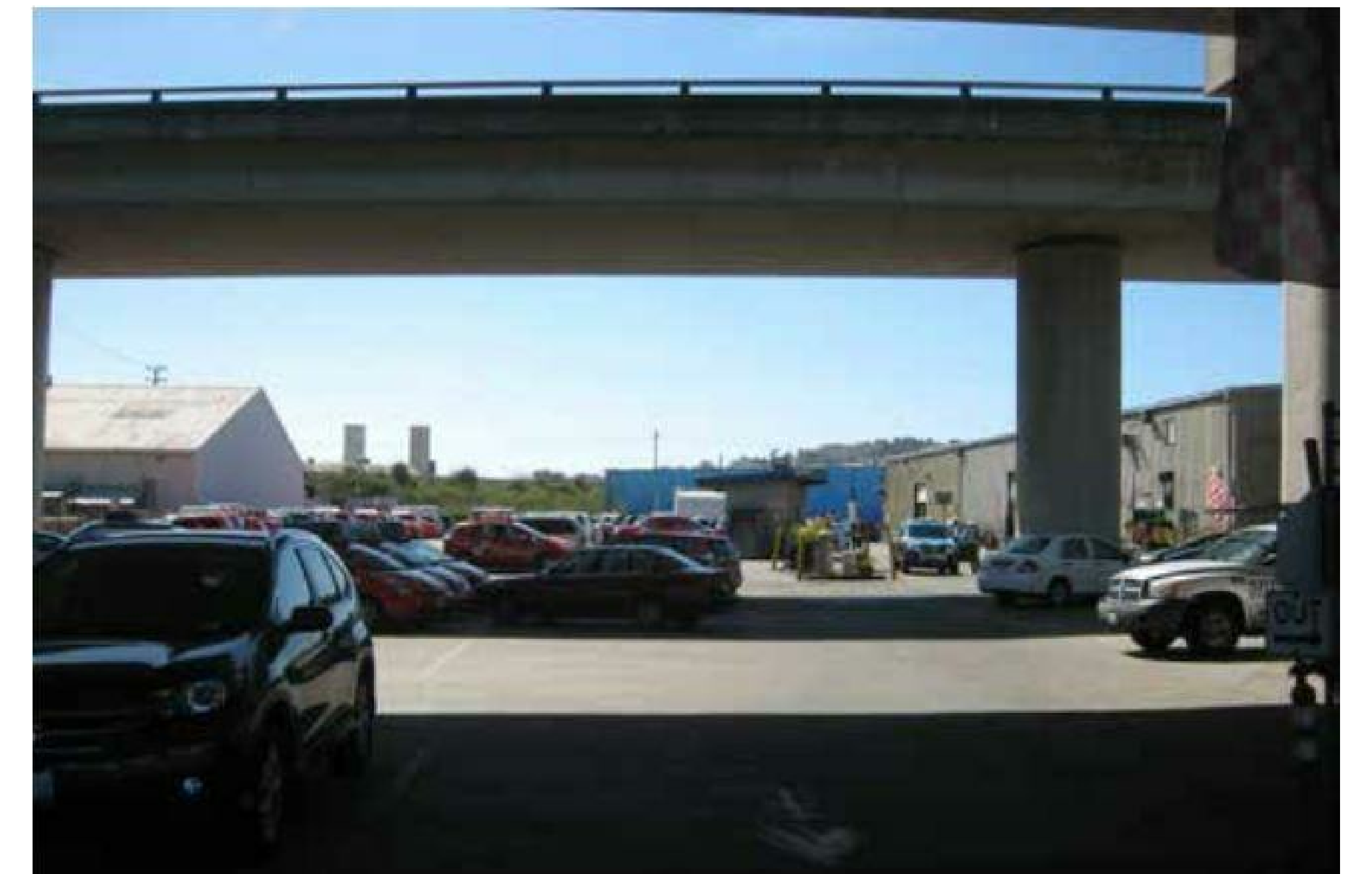
3 VIEW OF MAIN ENTRANCE INTO PROJECT SITE
