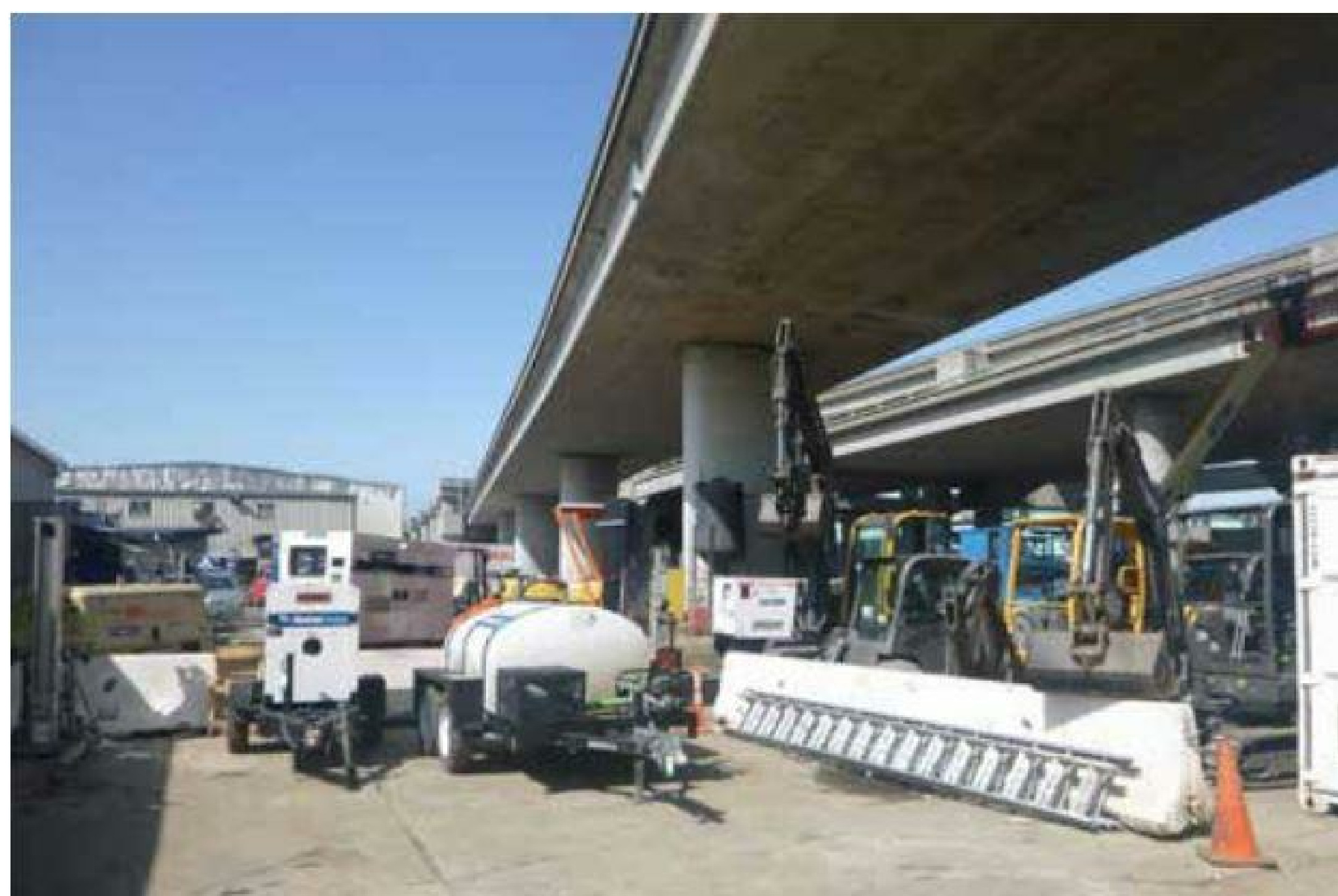
4 VIEW OF I-280 OVER PROJECT SITE
