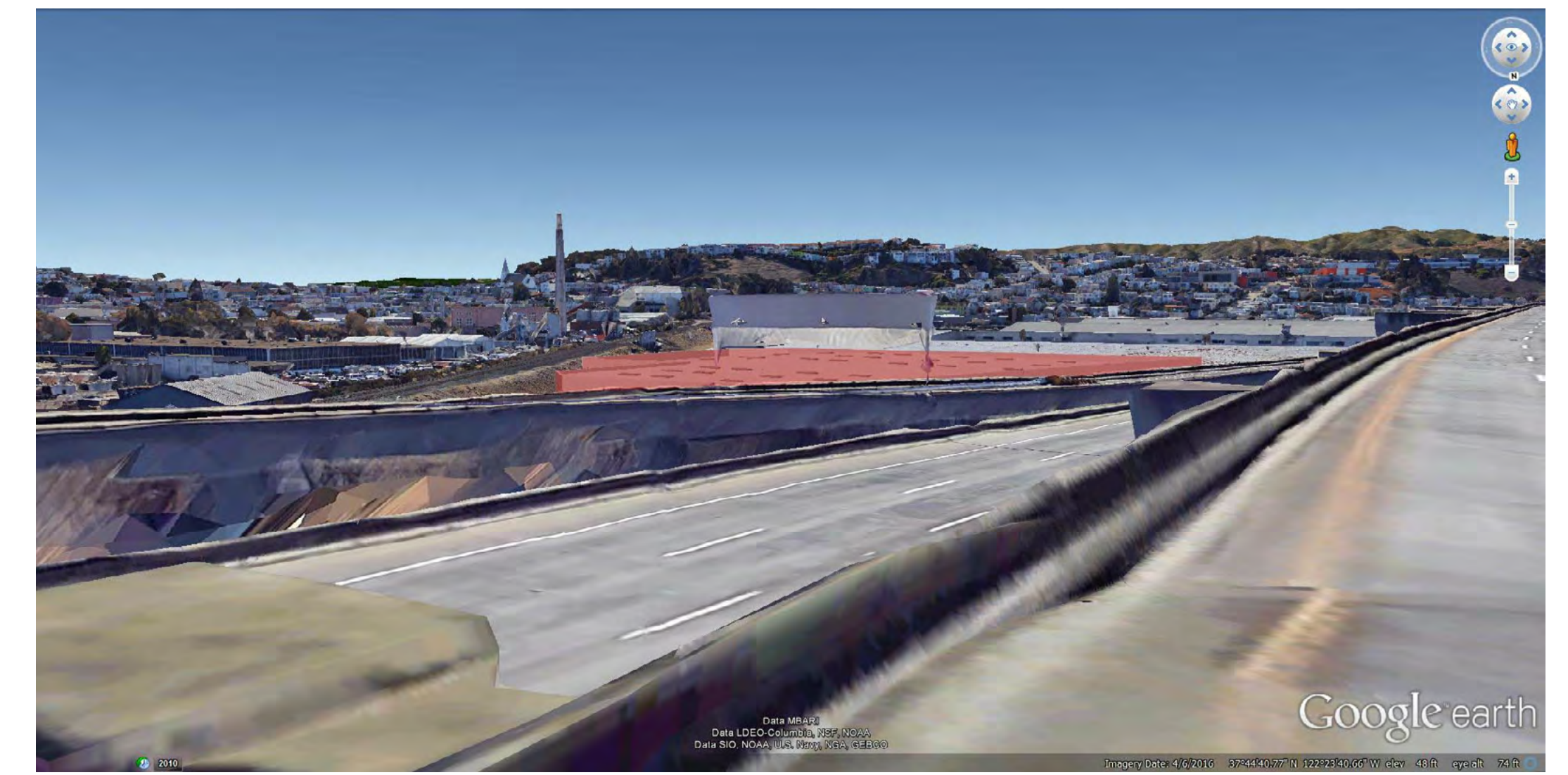
6 VIEW FROM I-280 SOUTHBOUND
