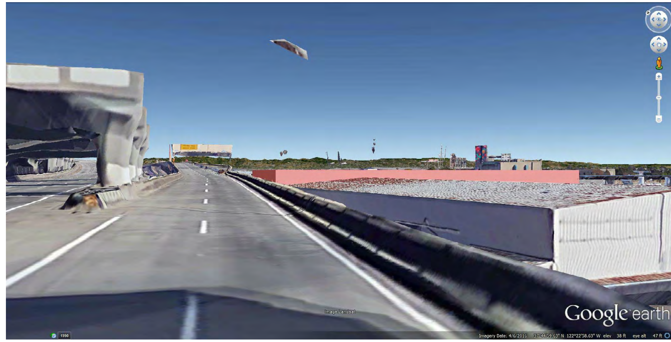
1 VIEW FROM I-280 - NORTHBOUND CESAR CHAVEZ EXIT RAMP
