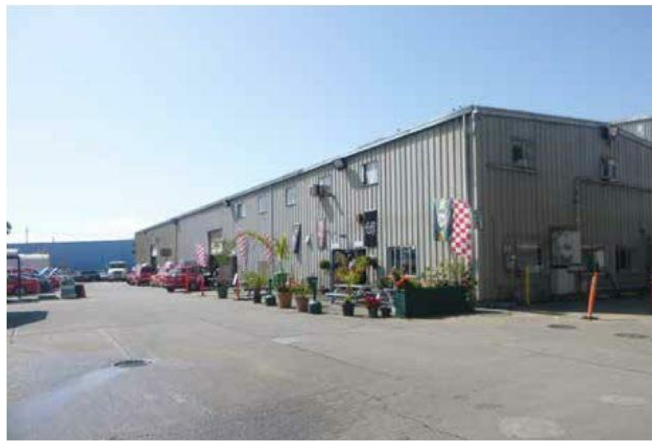
2 VIEW @ EXISTING BUILDING ALONG SOUTHERN SITE BOUNDARY LOOKING EAST
