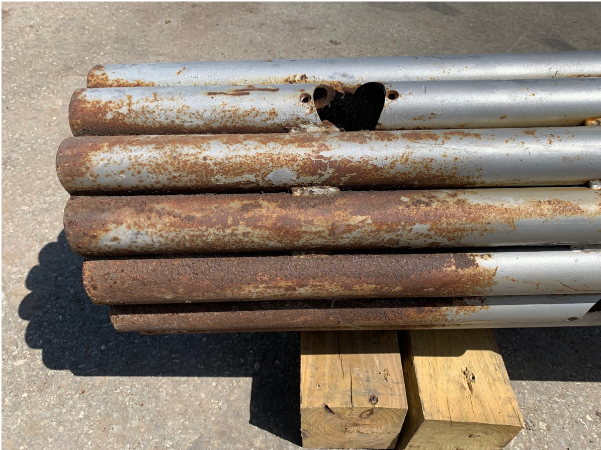
Bottom of the Sculpture Showing Advanced Ferrous Corrosion to Metal; Pitting, Blistering and Failure of Paint System
