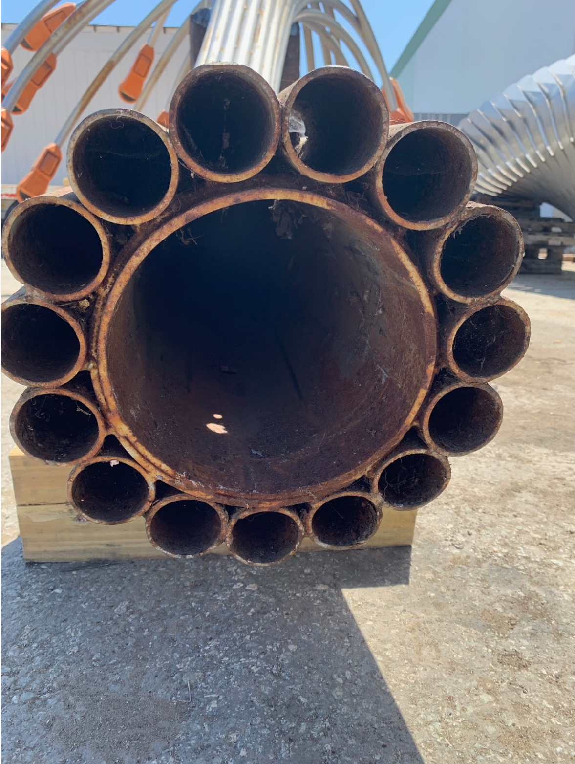
Interior View of Bottom End of the Sculpture Showing lack of Coatings and Extensive Corrosion
