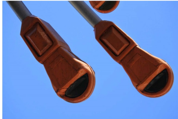
Detail of Parking Meter Heads. The once chartreuse colored glass now appears black, possibly from dirt inside the heads.
