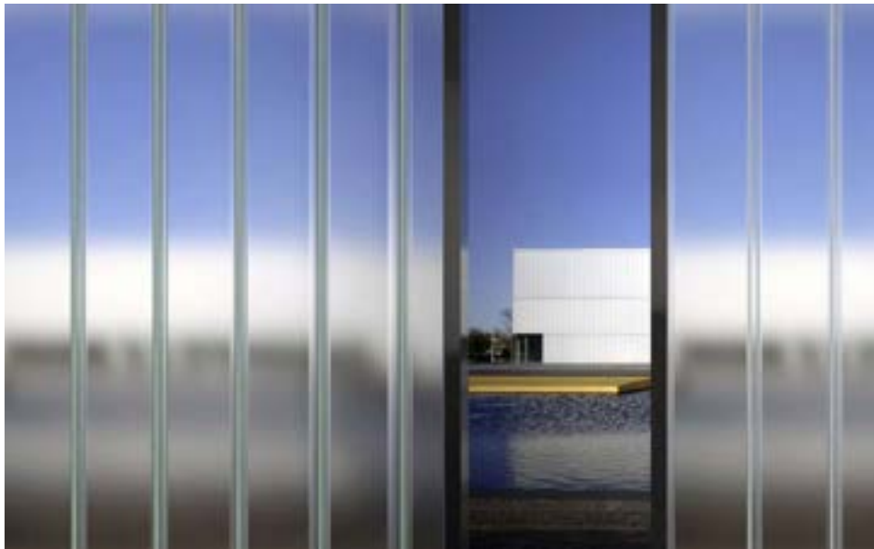
CHANNEL GLASS, NEW RESIDENCE AT THE SWISS EMBASSY, STEVEN HOLL, WASHINGTON D.C.
