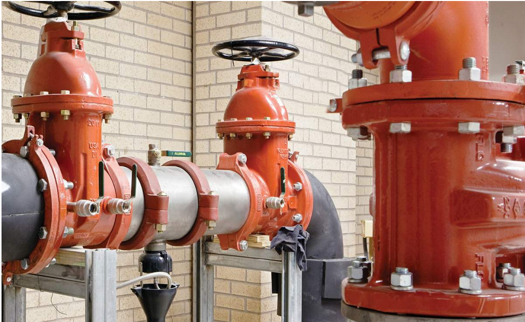
SUPPLEMENTAL FIRE WATER AIR GAP ASSEMBLY
