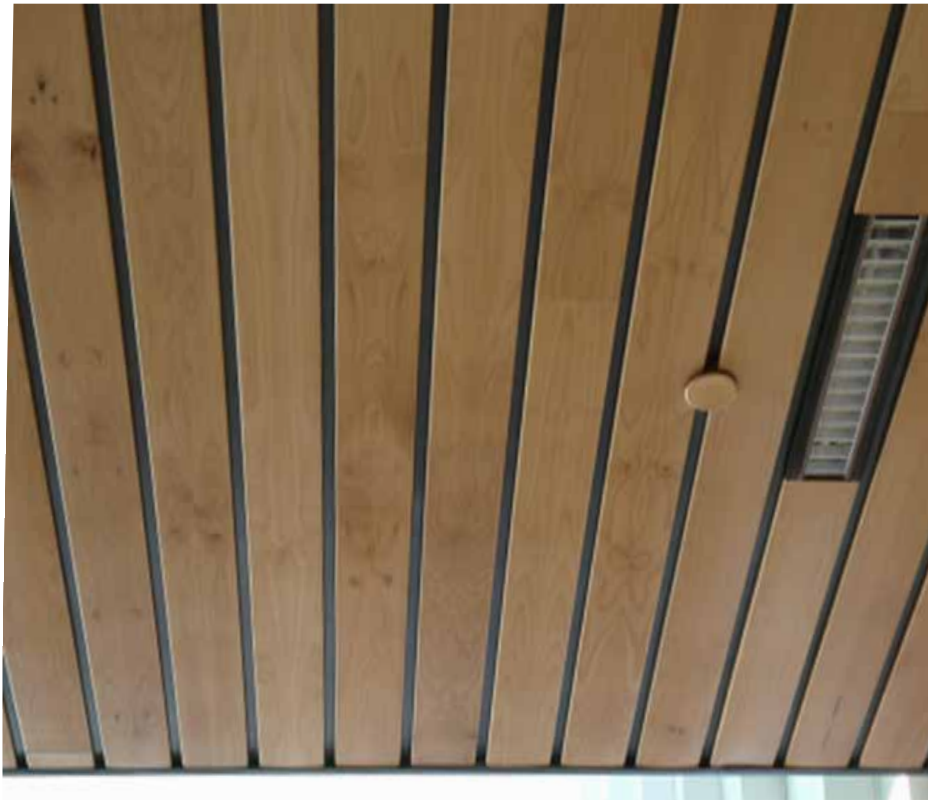
RESIN PRINTED ALUMINUM PANELS
